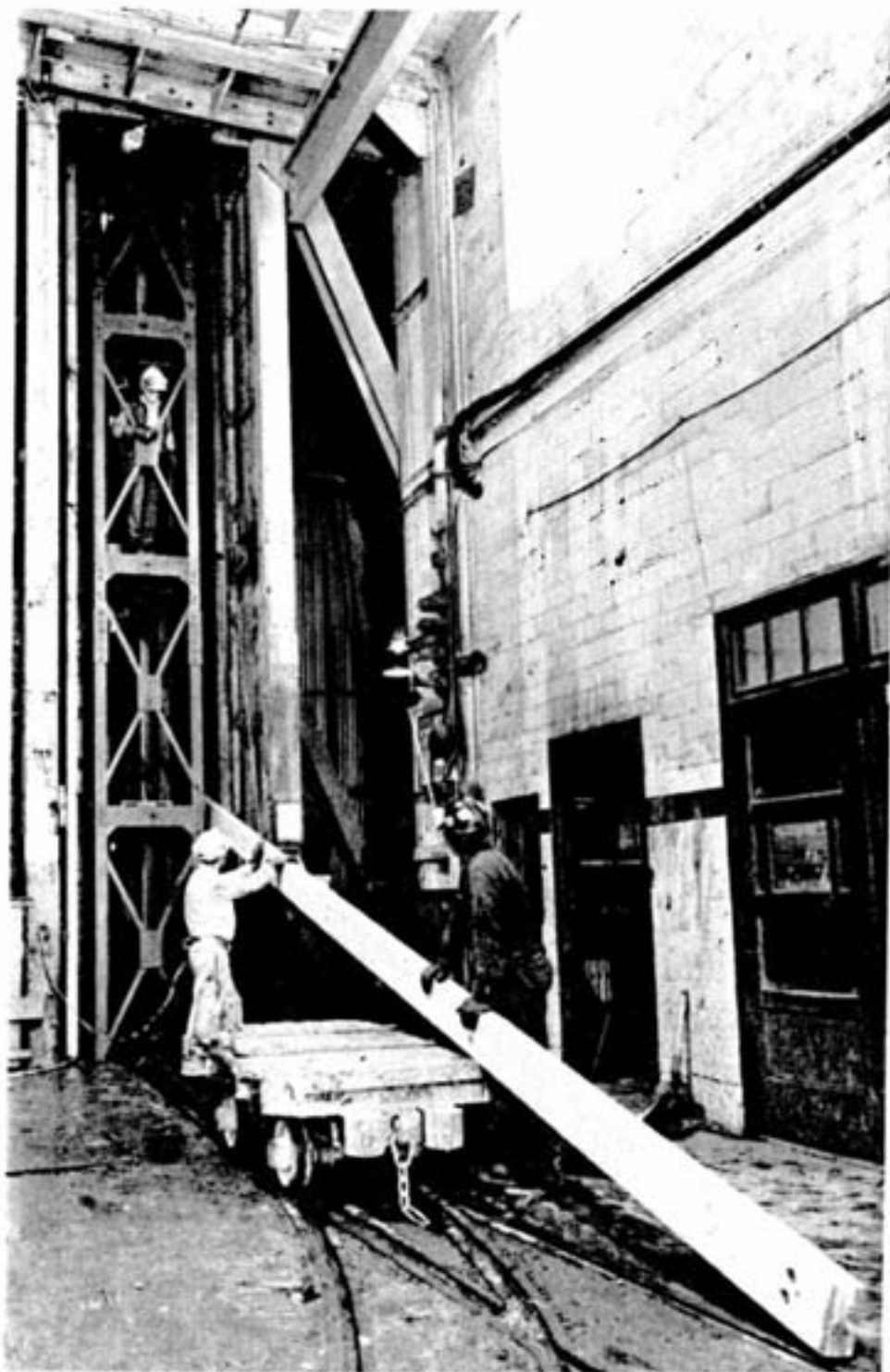
Henry Corcoran, operating shaft boss, front, and Wayne Desjardins are ready to help move a new shaft guide into the shaft. Gerald Turcotte stands in one of the several platforms of the new conveyance that makes guide replacement much easier.
