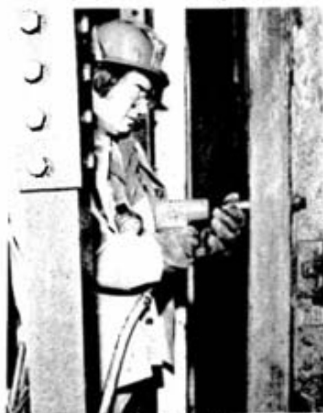
Ray Aubertine removes the bolt holding an old wooden guide in place.
