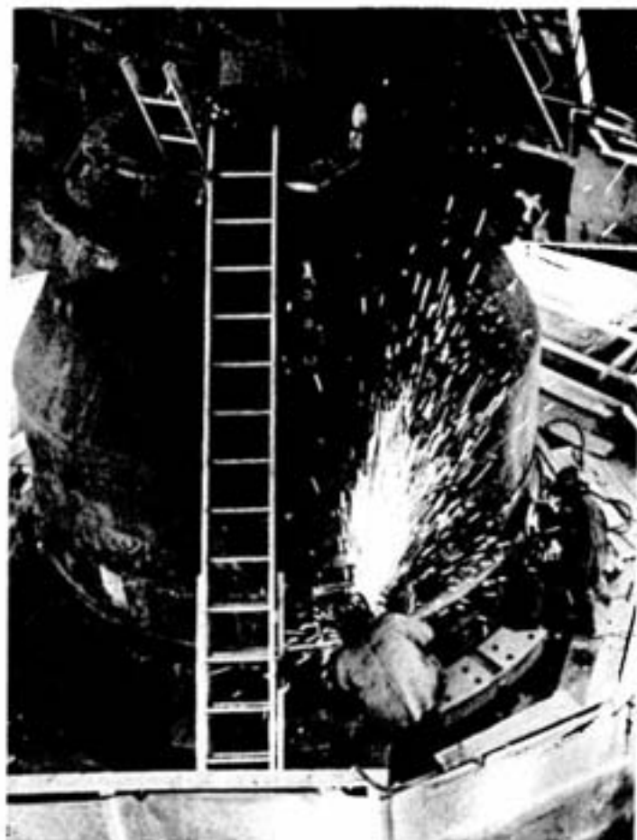
Roger Levesque, left, and Ed Whisset, send up a shower of sparks as they grind the surface of the TBRC.
