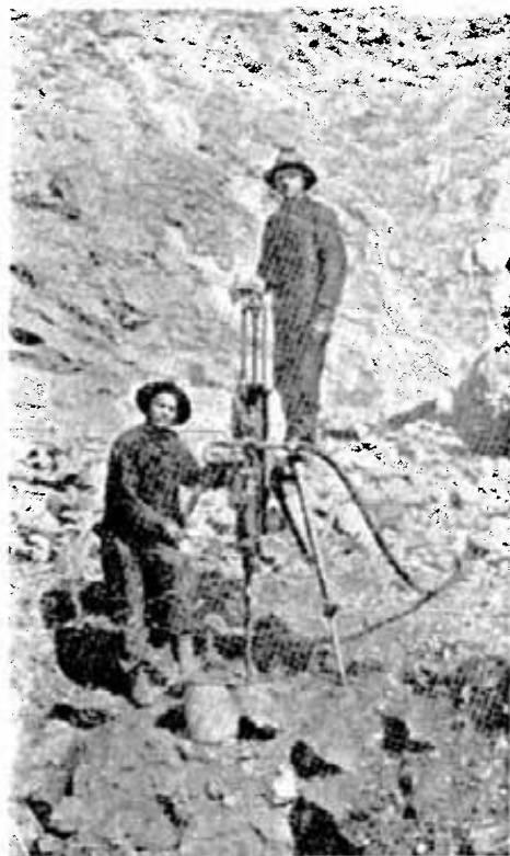
Taken about 1911, this photo shows Louis Marois, left, and his partner, L. Fera, manning one of the old piston drills in the open pit at Creighton mine. The machine was operated by compressed air and the steel was cranked into the drill hole by hand.
