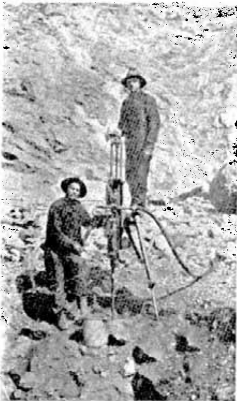
Taken about 1911, this photo shows Louis Marois, left, and his partner, L. Fera, manning one of the old piston drills in the open pit at Creighton mine. The machine was operated by compressed air and the steel was cranked into the drill hole by hand.
