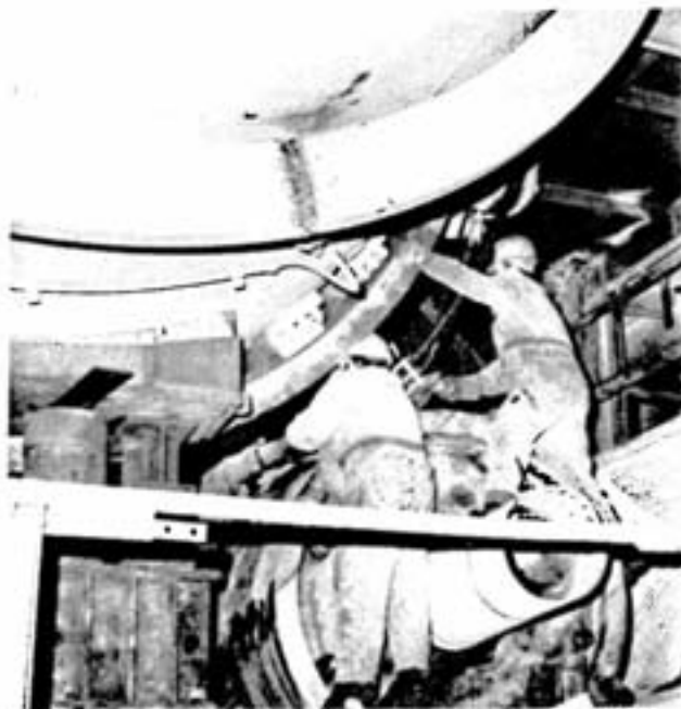
Maintenance mechanics Gino Oliver, left, and Henry Bazinet unhook the support trunnion from the Pettibone boom just before it is rolled into place under the roaster kiln.
