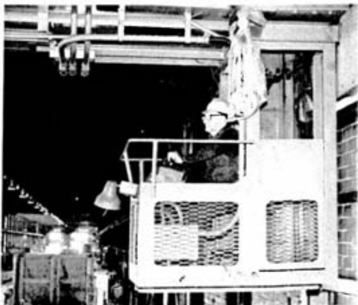
The addition of modern equipment usually leads to a more efficient operation with less manual labor involved. An example of this is the replacement of one of the cranes used to move nickel in the warehouse at the Port Colborne nickel refinery. Bob Conley is shown at the controls of the new Secord 5-ton crane. The S-crane's controls are easier to operate than the old one and the crane's movements are much smoother and safer.
