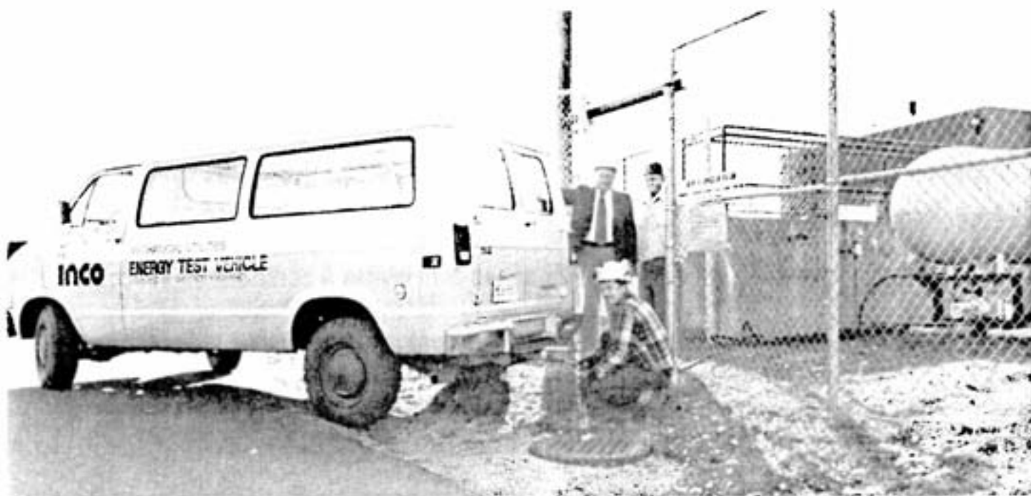
Propane is added to the van's pressurized fuel tank by Douglas Taylor while Alf Kaelas and Stan Rychlo look on.
