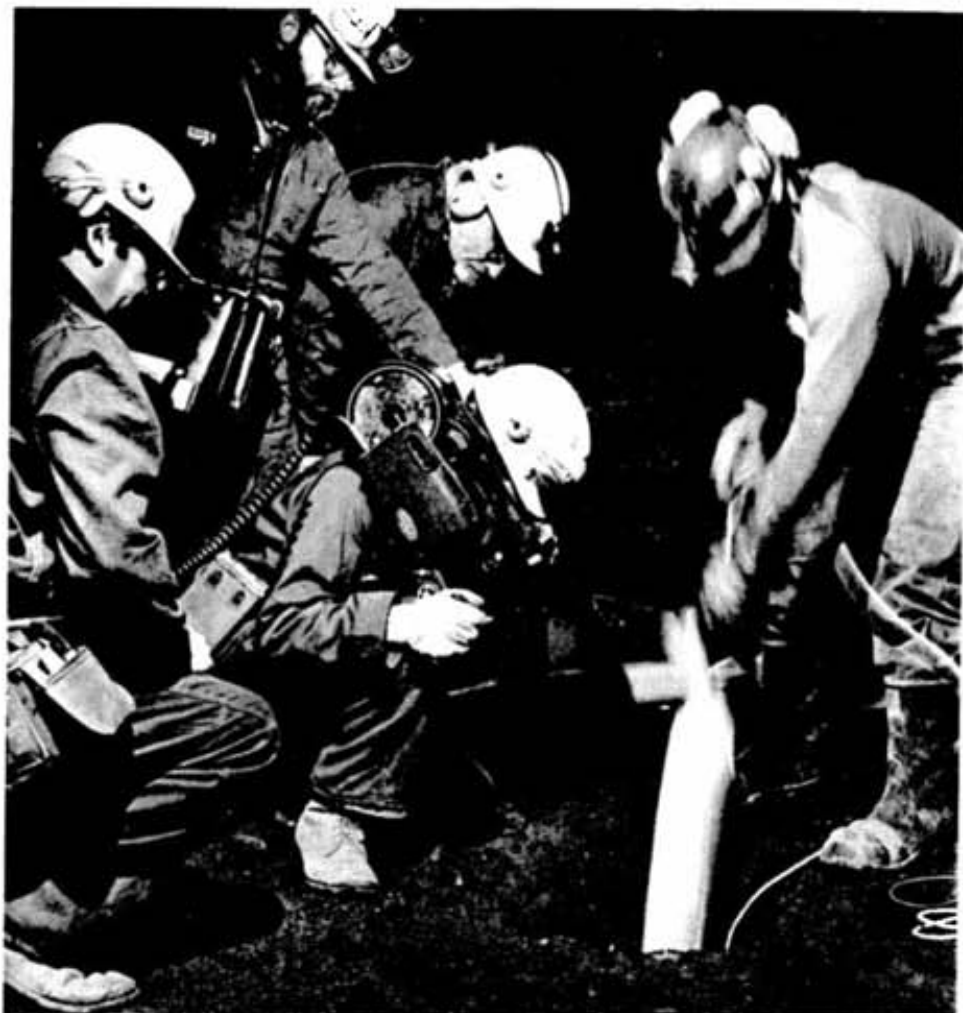
Film crews carefully follow a charge of Hydromex, an explosive, as it is lowered into the 6½-inch diameter blasthole.
