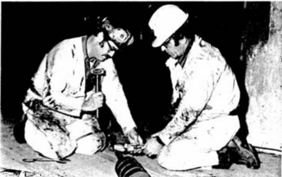
Preparing to cut the old rope to remove the attachment that connects to the cage are, from left, Armand Brideau, rigger first class, and Jerry Perrin, a rigger helper.
