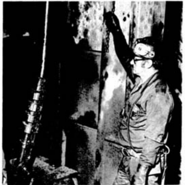
After connecting the new rope to the cage, John Komar, rigger first class, signals the hoistman to tighten the rope.
