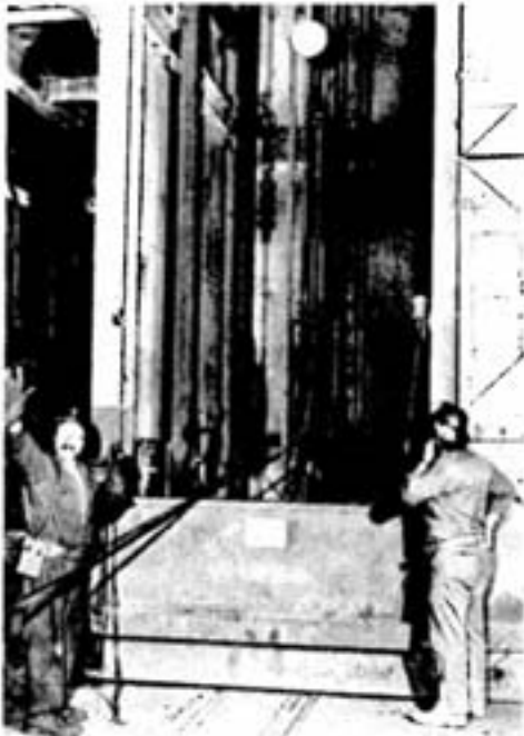
Ron Benoit, rigger first class, signals the winder operator to begin winding the old rope onto the reel as it is being removed from the shaft. Looking on is Donald Pierce, general foreman, operating and maintenance.
