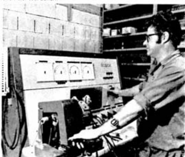
Gerry Barnett, garage mechanic, keeps a close eye on readings at the alternator test bench.
