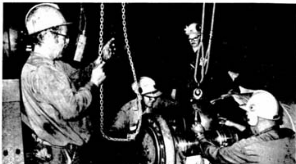
Positioning the top bearing cap of the No. 2 skip hoist generator are, from left, Don Golloher, second-class garage mechanic, Jim Pentney, first-class rigger, Don Stephens, maintenance foreman, and Barry Van Horne, first-class maintenance mechanic.
