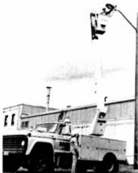
Servicing one of Little Stobie mine's mercury vapor light standards is a breeze for linemen Jay Connors and John Kelly . Here John stands comfortably and safely in the fibreglass bucket of the Inco bucket truck. With controls at the top as well as at the bottom of the boom, he can easily work as a one-man crew. Speed, efficiency and safety are some of the benefits enjoyed through the use of these versatile vehicles.
