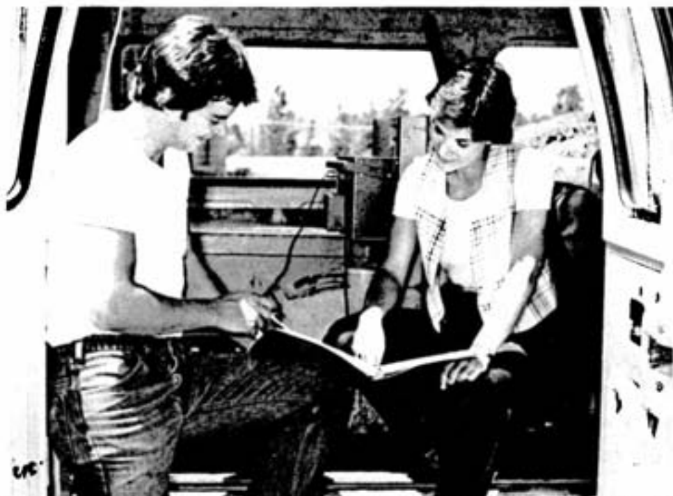
Inco environmental analysts Barry Bissonnette and Elizabeth Minard are checking a readout from the mobile SO 2 monitor, mounted in this environmental control van. The monitor is used to verify predictions made concerning ground level SO 2 concentrations from the superstack and the IORP chimney. These readings aid Inco's environmental control department in refining the dispersion formulas. The unit, stationed in Copper Cliff, operates within a 20 kilometer radius.
