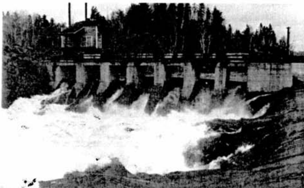
Water flows through spillway at Nairn plant
