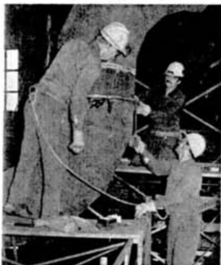
Because of age, two waste heat boilers in the anode department of the Port Colborne nickel refinery had to be rated for lower maximum pressure during the past few years. Finally, they had reached a point where they could no longer operate effectively, and it was decided to replace them. Cost of the project will be $3.8 million by the time it is complete in September. Above, from left, ironworkers Lyle McCutcheon , Dave Roberts and Roger Jacques assemble some ductwork on number two furnace.
