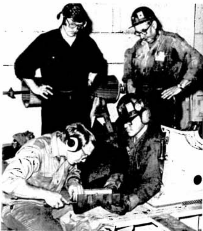
Standing, Terry Exworth, left, and Gary Judson watch while Stan Ojanpera, left, and rigger Wayne Lamore scrape the speed increaser bearing.
