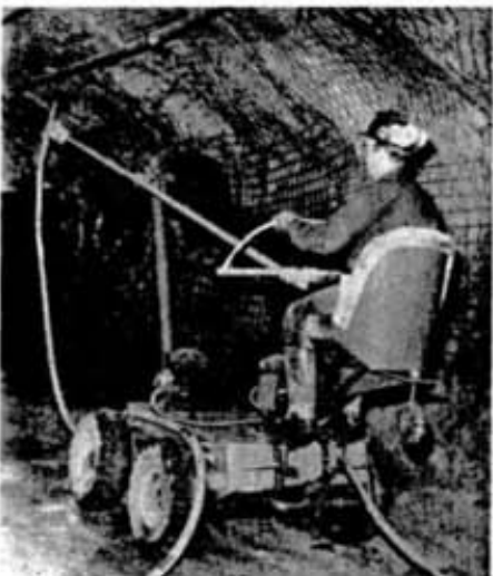
Developed by Copper Cliff South mine personnel, this longhole drill carriage was modified and adapted to remotely hold a shotcrete nozzle away from the operator and so remove him from dust and back spray while shotcreting walls and roofs underground. The unit comes complete with two air-driven traction motors.
