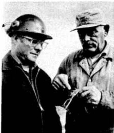
That's Carlo Scopazzi , right, a track boss with the Copper Cliff track maintenance section, displaying the damage to his prescription safety glasses to foreman Joe Longhi . Recently, while hitting a track spike with a track hammer during track repairs in the slag dump area, a piece of steel flew from the spike and struck the lens of Carlo's spectacles. The incident caused no injury to the eye. Subsequently, Carlo recently was enrolled in the Wise Owl Club of Canada.
