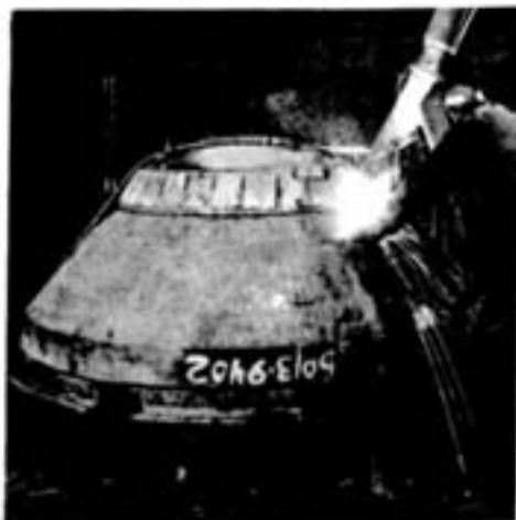
In order to increase wear life, second-class welder Victor Naumenko welds wear pads on a shorthaul locking nut in a repair area at Frood-Stobie mill's crushing plant. The task is part of a rebuild for the locking nut on a shorthaul crusher mantle.
