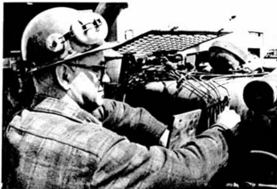
First class garage mechanic Morris Page adjusts the bracket holding fuel injection lines for an ST-2 scooptram, in for a general overhaul from Garson mine.
