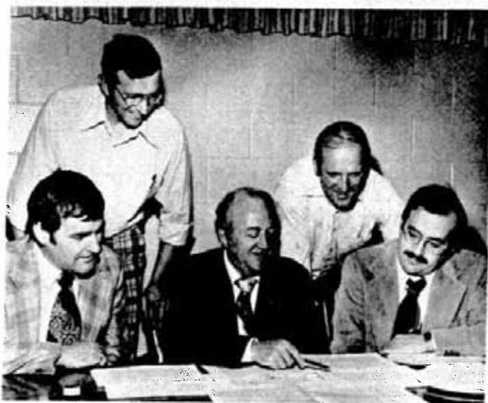
Inspecting the final results of the air measurement survey are, from left, Claude Kerr, senior field engineer; Bob Todd, industrial evaluator; Gerry Cullain, manager, utilities; Allan Uildersma, hydraulics technician, and Berno Wenzl, energy management co-ordinator.
