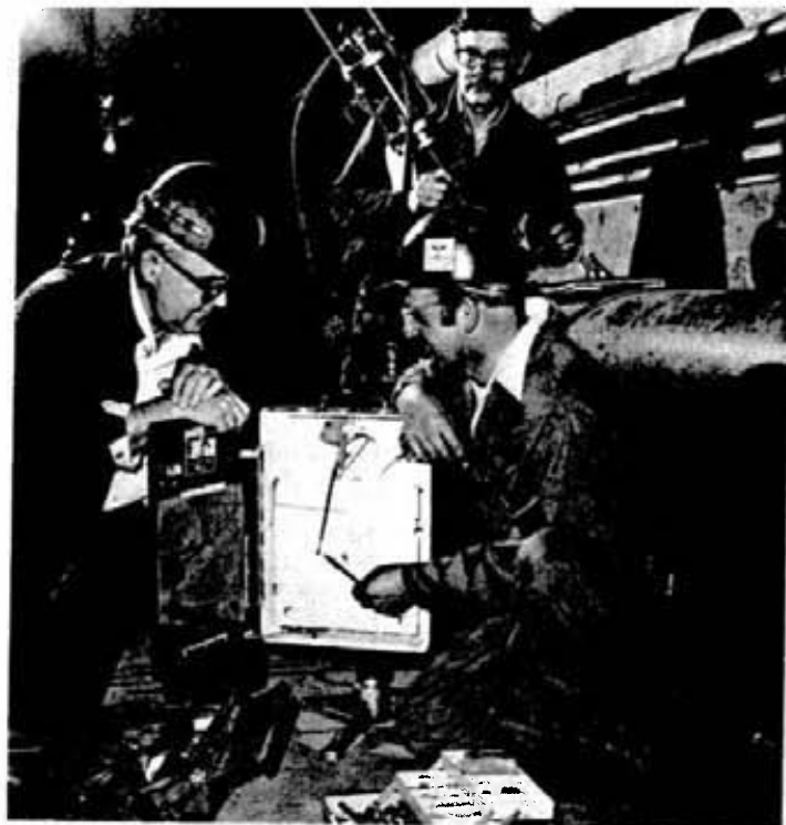
In the Levack compressor building services tunnel, a flow recorder is examined to determine output of the compressors. Checking the recorder are, from left, Lew Butler, supervisor of utilities for the Levack complex, Eero Mansikka, senior surveyor with central utilities, and, kneeling, Allan Uildersma, hydraulics technician, central utilities department.
