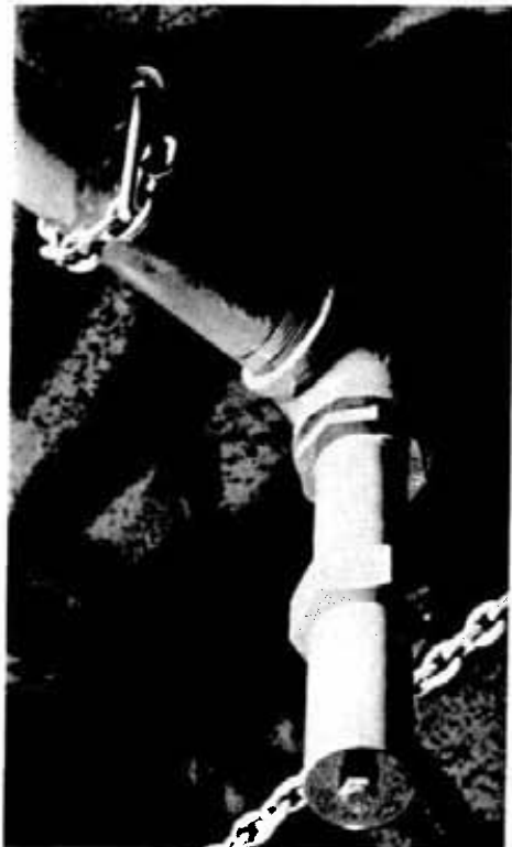
Centrally located overhead, this discharge nozzle, when activated, emits the Halon gas.
