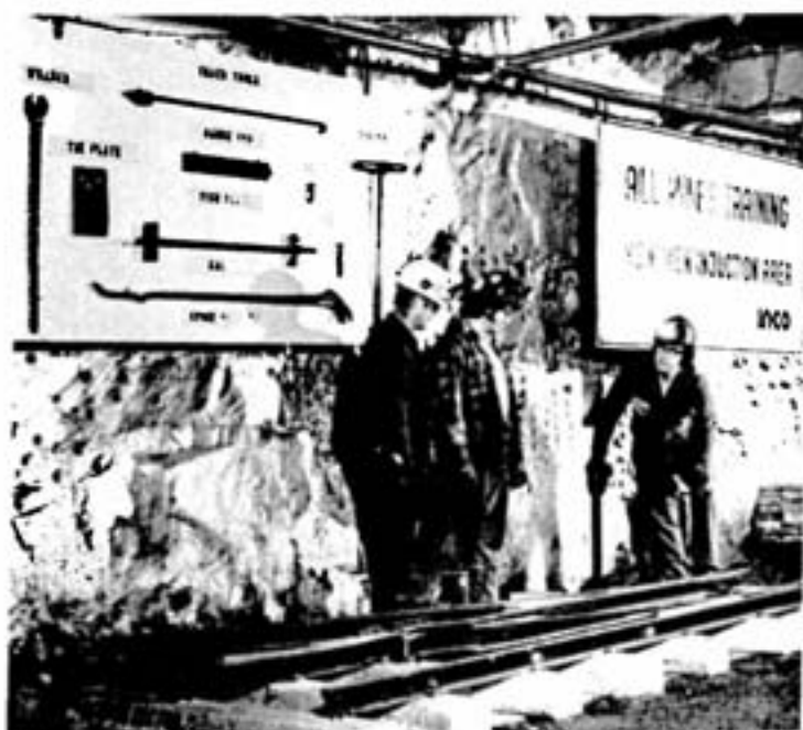
Trainees Jim Harrison, left, and Keith Griffith listen and watch while instructor Yvan Forgues explains the operation of a switch throw on underground tracks.
