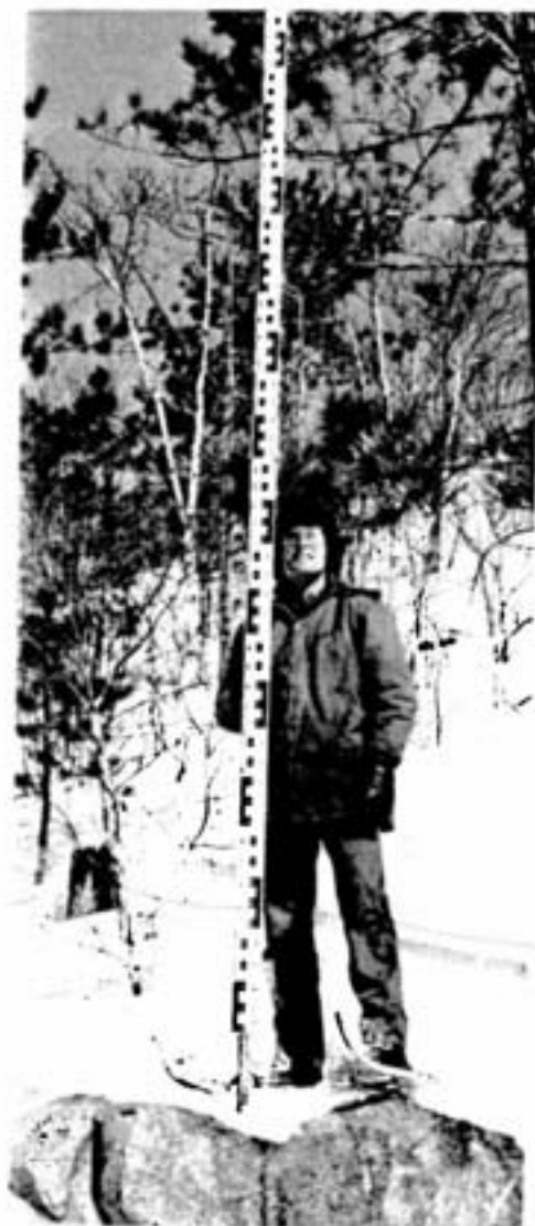
At a survey site, Jim Swain, survey assistant, is holding a reading from a level rod at a bench mark.
