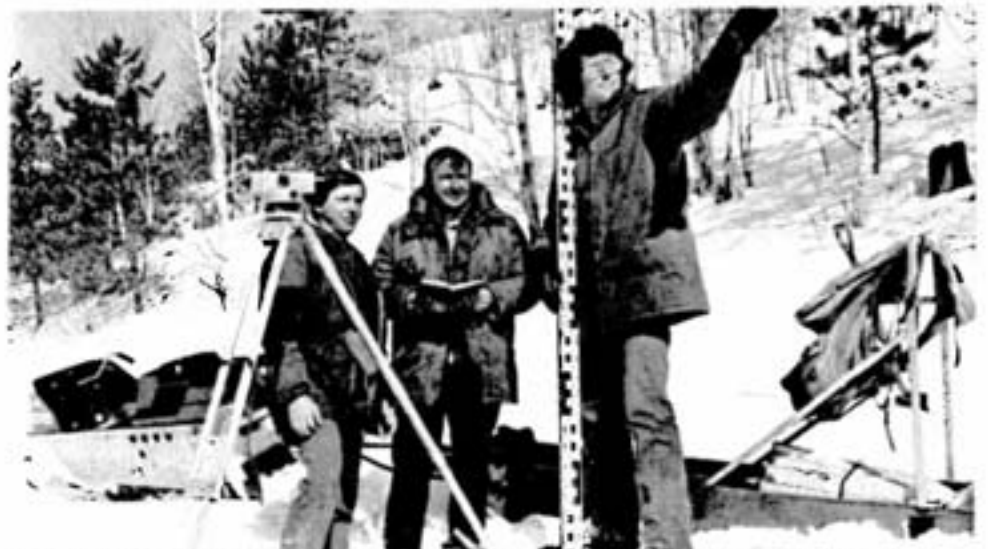
Preparing to establish elevations of bench marks by using a precise level and a leveling rod are, from left, instrumentman Bob Hicks, instrumentman Gord Pedersen, and survey assistant Jim Swain.
