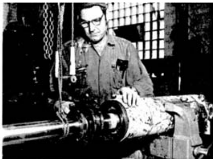
In preparation for repair work, first class maintenance mechanic Reg Lalonde removes the rod assembly from an ST2A hoist cylinder.
