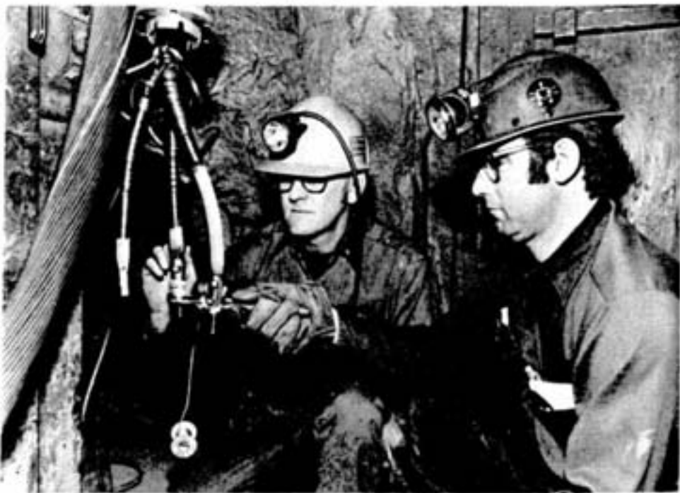
Completing a program begun in 1976, first-class electricians Fred Wright , left, and Mark Pennarun splice a new mine shaft power cable running from surface to the 2200 level of Copper Cliff North mine. The additional power supply is designed to provide for increased electrical consumption in the lower levels of the mine.
