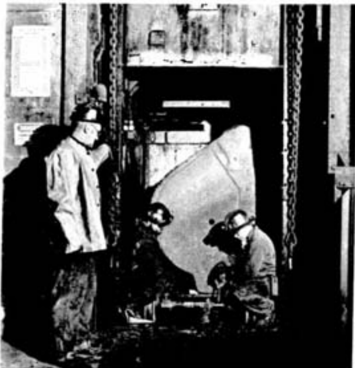
Cage tender Raymond Bouchard, left, waits while Eddi Graham, drill fitter, and Dieter Rothe, second-class rigger, secure a five-yard bucket onto a lowbed truck in the cage for hoisting to surface.
