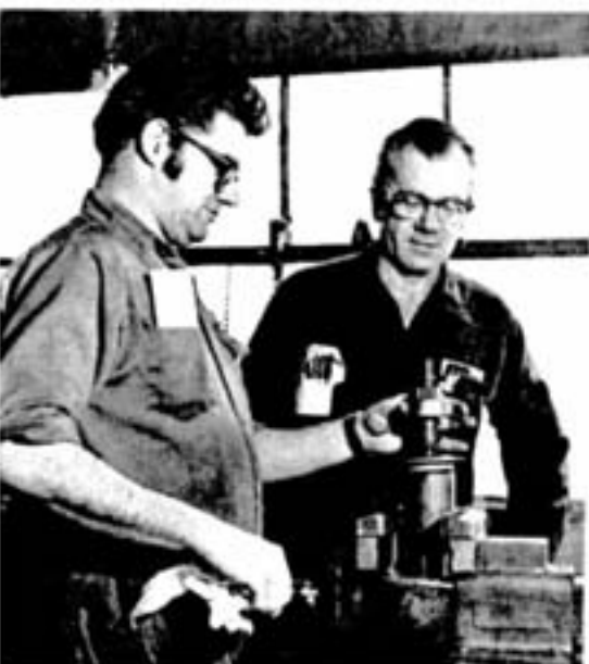
First-class garage mechanic Gerry Barnett, left, and garage mechanic leader Alex Dure repair a Bosch starter.
