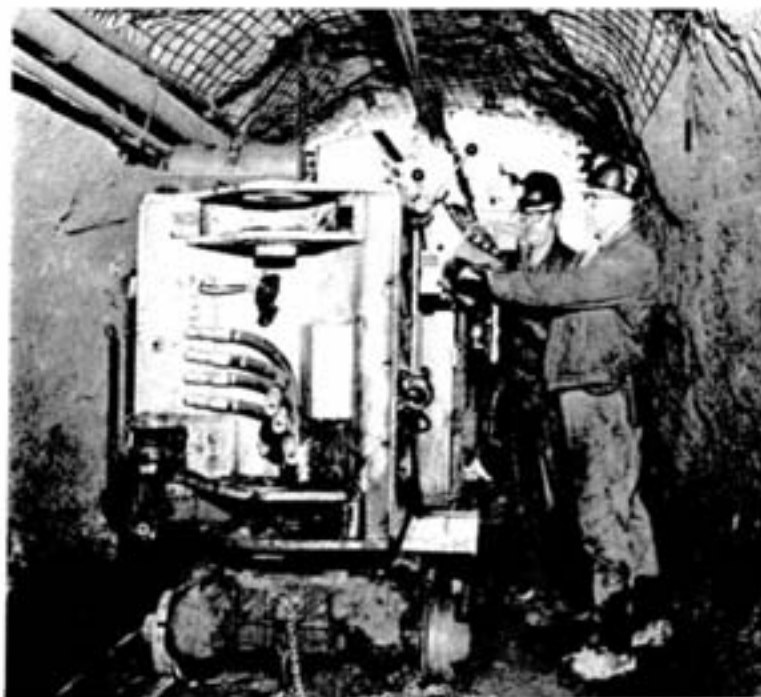
In the main south drift at 1200 level, rigger helper John Dutresne, left, and Henry Prinoski, rigger leader, inspect the chassis on a bunk truck to ensure that it's properly secured before moving it to the shaft station and then to surface by cage.
