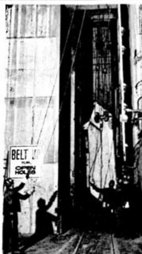
How do you move a 26-ton capacity steel box, originally fitted on a haulage truck, from surface to the 1500-foot level underground? Add to this the fact that the box itself weighs 6 tons and is cumbersome to handle! Nothing to it, according to the Copper Cliff South mine rigging crew who successfully lowered the unit down the mine shaft with only one inch clearance. That's teamwork!
