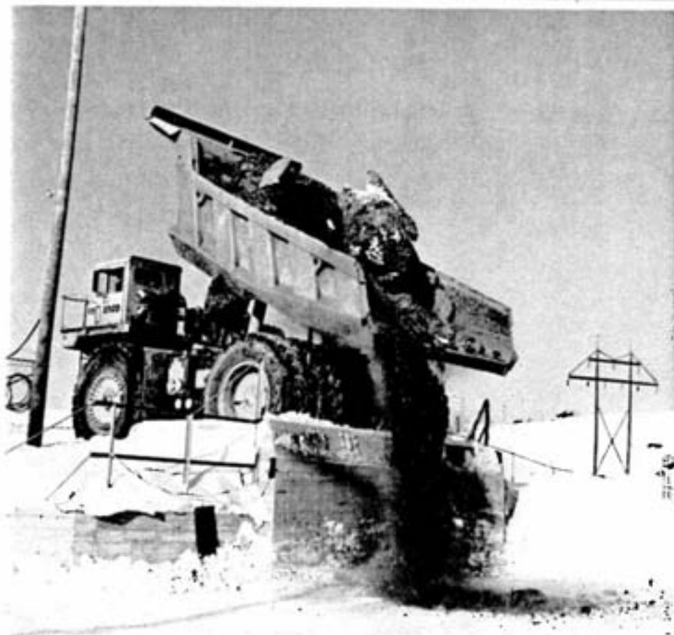
The first 75-ton load of rock for Copper Cliff South mine's 826.0 rockpass and 830.0 orebody was recently dumped by haulage truck driver Harvey Winn . The rockpass extends from surface near Highway 17 west to the 1000 level; from there, the rock will be picked up and dumped into the designated stopes.
