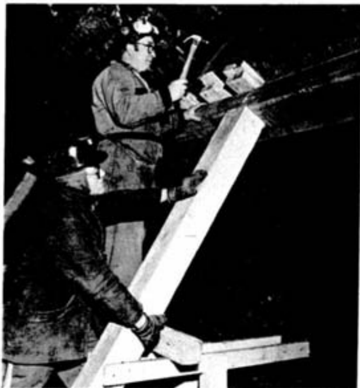
Shoring the remaining brick during a repair of the number one stretch converter are second-class carpenters Raymond Dicaire, left, and Angelo Dirocco.
