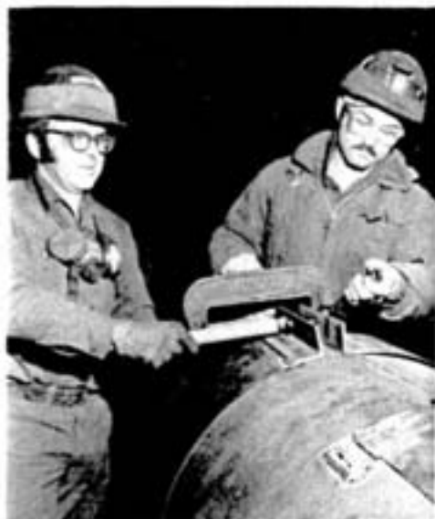
First and second-class maintenance mechanics Rolly Landry, left, and David Violette band an offtake pipe.
