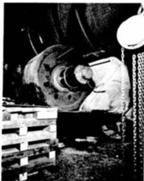
When workmen at the Iron Ore Recovery Plant noticed a crack in one of the large rollers supporting the No. 5 reducing kiln, plans were made to remove the 67-inch diameter roller and to install a spare assembly. Normal procedure is to remove the weight of the kiln from the rollers, utilizing two 350-ton jacks and then exchange the broken roller with a new one, using a crane. Due to very limited access and headroom, a crane could not be used. Consequently, thanks to the excellent co-operation from personnel at Creighton and Copper Cliff South mines, the lifts were carried out safely and in record time with the help of an ST8 scooptram which eliminated extensive rigging to remove the 13-ton rollers. At left, the scooptram is in position under the kiln where maintenance mechanics assist in placing the roller into the scoop bucket. The photograph at right shows the men and equipment involved in the move. Kneeling, from left, Gino Oliver , Cliff Boomhower and Marco Urso . Standing, from left, general foreman Ilario Toniolo , Dale Gutjahr , Ray Forcier , Bill Mirult , Marcel Poulin and foreman Vic Riutta .
