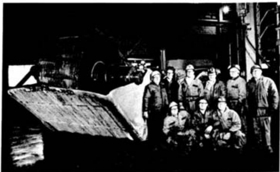
When workmen at the Iron Ore Recovery Plant noticed a crack in one of the large rollers supporting the No. 5 reducing kiln, plans were made to remove the 67-inch diameter roller and to install a spare assembly. Normal procedure is to remove the weight of the kiln from the rollers, utilizing two 350-ton jacks and then exchange the broken roller with a new one, using a crane. Due to very limited access and headroom, a crane could not be used. Consequently, thanks to the excellent co-operation from personnel at Creighton and Copper Cliff South mines, the lifts were carried out safely and in record time with the help of an ST8 scooptram which eliminated extensive rigging to remove the 13-ton rollers. At left, the scooptram is in position under the kiln where maintenance mechanics assist in placing the roller into the scoop bucket. The photograph at right shows the men and equipment involved in the move. Kneeling, from left, Gino Oliver , Cliff Boomhower and Marco Urso . Standing, from left, general foreman Ilario Toniolo , Dale Gutjahr , Ray Forcier , Bill Mirult , Marcel Poulin and foreman Vic Riutta .
