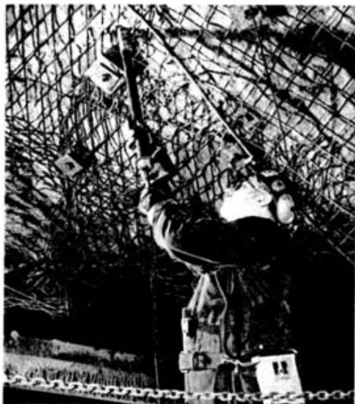
Introduction of the cable bolt is complete and now the grout plug is being placed in the collar of the hole by longhole driller Dan Sakovic. The plastic breather tube has been placed through the grout plug, and the hole is now ready to be sealed.
