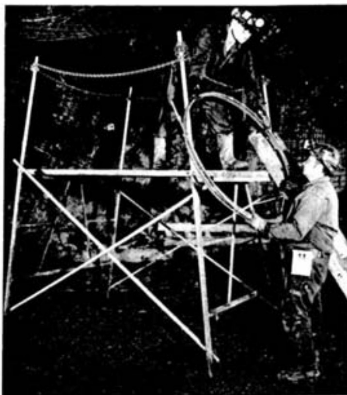
The new uphole cable bolting technique features portability, simplicity, and increased safety. Longhole drillers Dan Sakovic, left, and Gabe Bisailon prepare to insert the new lightweight \frac{3}{8} -inch cable into previously-drilled holes.
