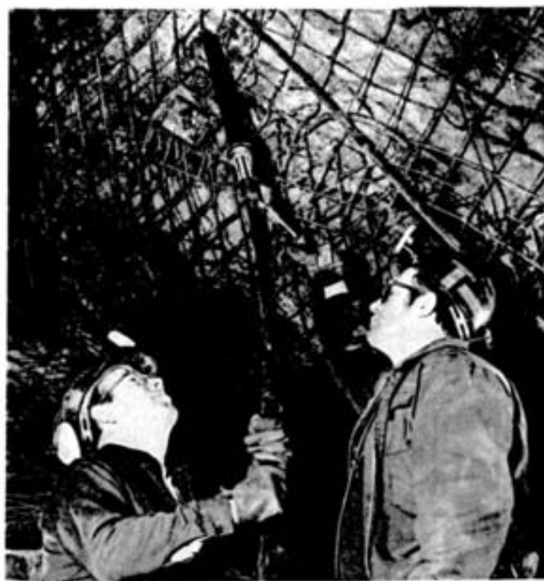
Mine planner Fred Birchall, left, and Gabe Bisaillon, longhole driller, tighten the nut at the lower end of the grout plug to seal the hole. The bottom of the grout plug is now attached to a one-inch-diameter plastic grout hose.
