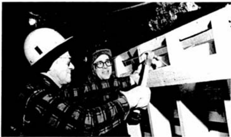
inside the number one stretch converter at the Copper Cliff smelter, Dick Began, left, second-class carpenter, and Jerry Lockman, carpenter apprentice, install backforms to hold brick in place during a repair of the converter.
