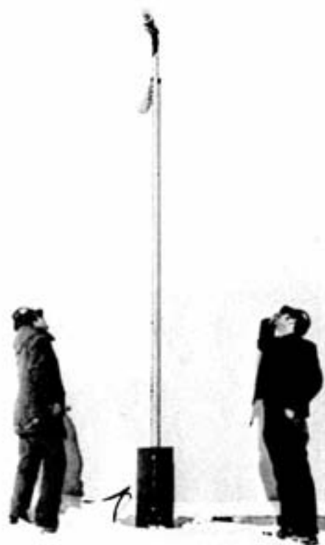
Members of the Copper Cliff maintenance field force recently installed some 20 low-pressure sodium lamps around the base of the 16-million gallon capacity water tank in Copper Cliff. The light-sensored lamps turn on and off automatically at dusk and daybreak. Above, Dan O'Reilly , left, and Mike Demers , both first-class electricians, inspect one of the new light fixtures. Below, Mike Beers , left, a fourth-year apprentice, watches Art Leroux , first-class electrician, as he works on one of the junction boxes.
