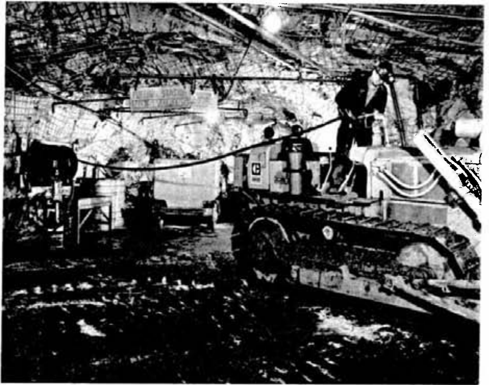
Loading a bulldozer from the hydraulic tanker at the loading station on the 1500 level is 'dozer operator Nick Perih.
