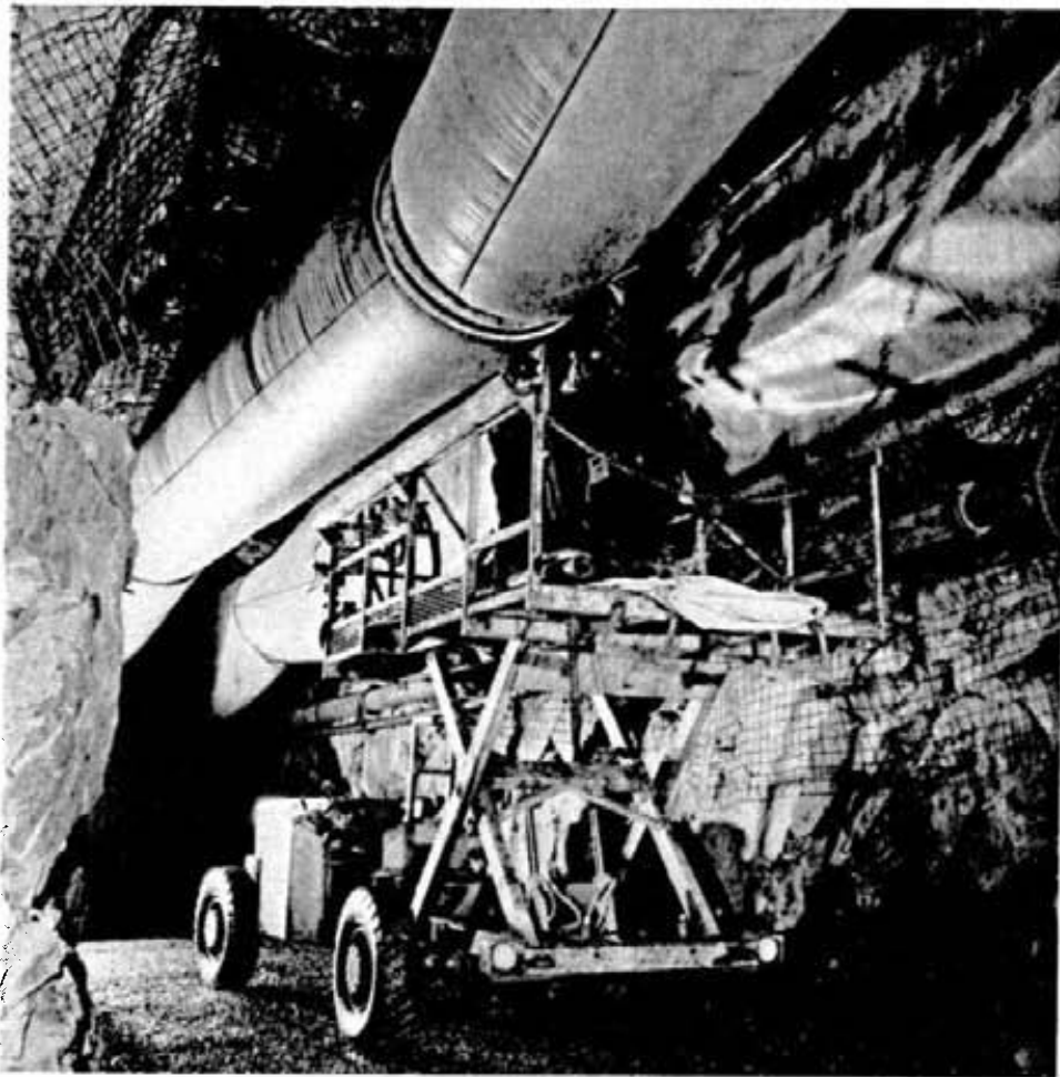
Installing flexible ventilation tubing on the 1500 level of Copper Cliff South mine are jumbo drillers Fred Elliott , left, and Jim Plummer . Compared to conventional vent ducting, the flexible tubing offers increased safety and easier handling during installation. It also shows significant cost advantages in handling, installation time and initial purchase.
