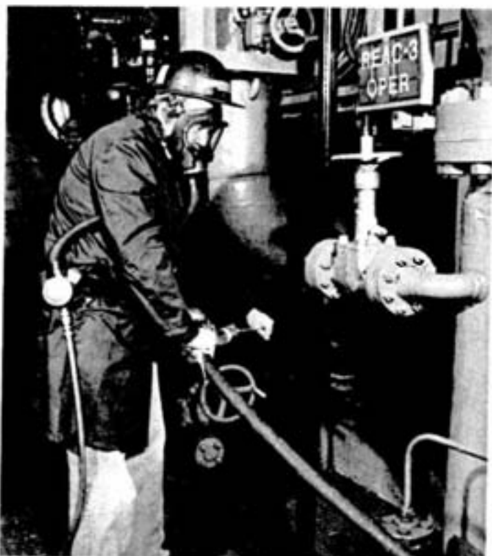
While collecting gas samples for content analysis, "Hilly" Gilchrist, process assistant at the nickel refinery, wears a breathing air mask which receives air from the IPC plant's breathing air system manifold.
