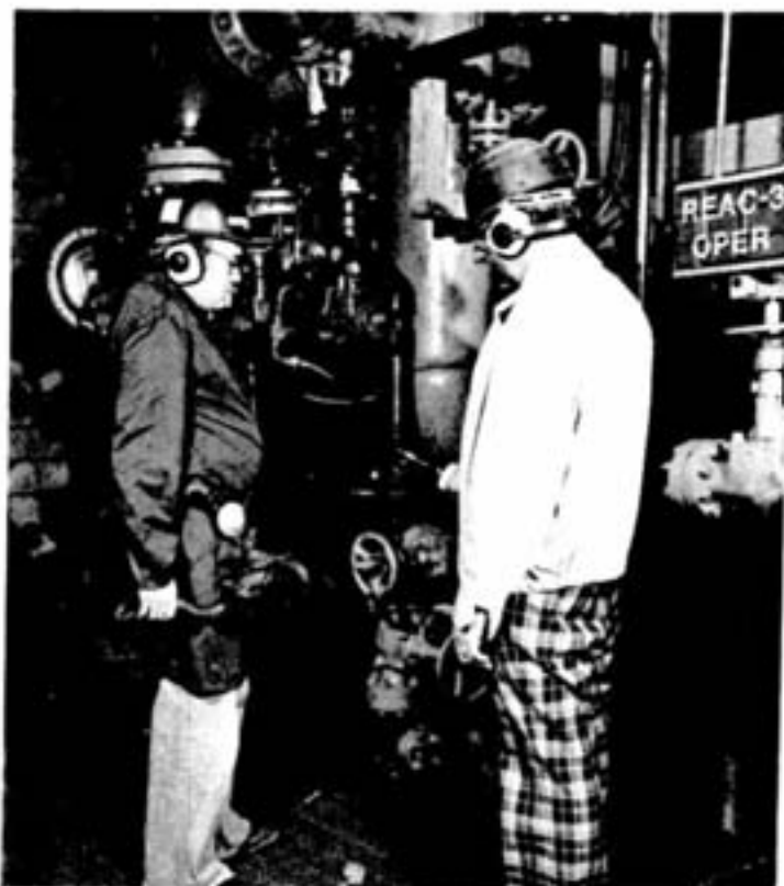
At the IPC plant's No. 3 reactor, "Hilly" Gilchrist, left, and Harvey Gere, safety supervisor, Copper Cliff nickel refinery, review leak-checking procedures, using a propane torch.
