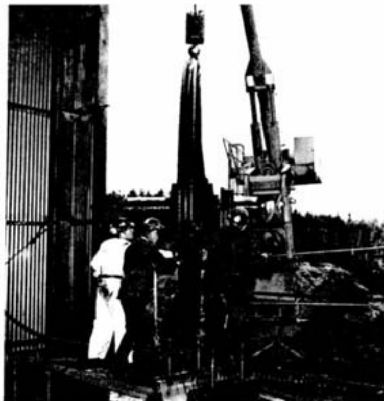
Guiding the sheave as the crane operator removes it from the headframe are, from left, Sinclair MacKenzie, first class rigger, Roger Savourin, plater, and Ken Taylor, first class rigger.
