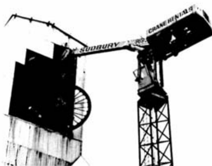
At the top of Levack mine's No. 2 shaft headframe, the operator of the special crane has a perfect view of his target and can easily maneuver the old sheave wheels out and down.
