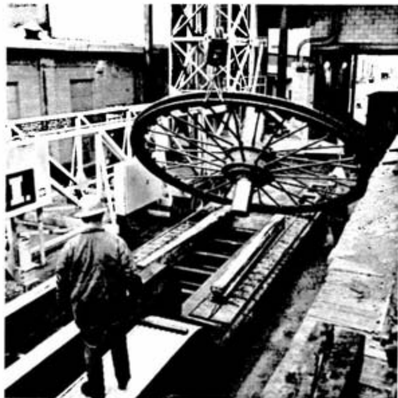
With the help of a 30-ton telescoping crane, Ray Cormier, left, and Martin Nowoselsky, both first class riggers, gently ease an old sheave wheel onto a waiting flatbed truck.
