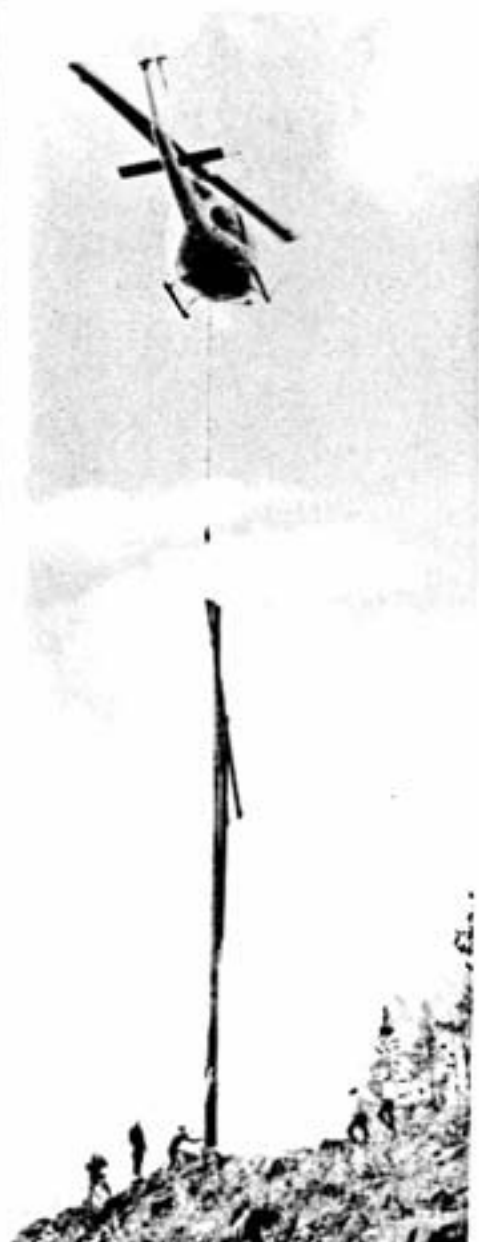
Power poles are carefully lowered into position. The pole-setting crew was led by Gary Guy, PowerTel foreman for the project
