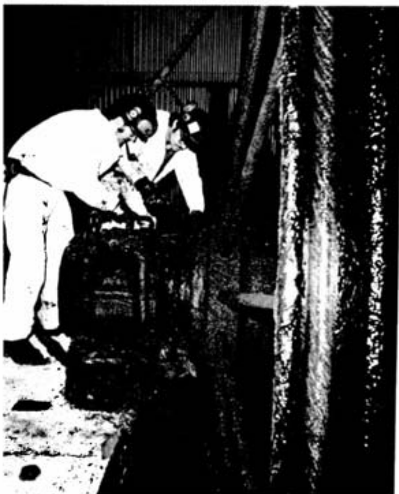
Ron Marcotte, left, first class maintenance mechanic and Claude Gravel, first class machinist, dismantle the sheave wheel bearing cap to allow removal of the 14-foot-diameter wheel.
