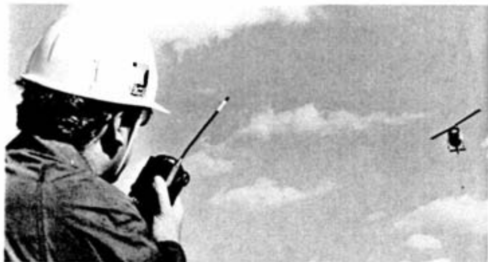
Clary Gatien, president of PowerTel Utilities, is in constant ground-to-air communication with the helicopter being used to install the powerline poles. Here the chopper is returning from the work site to pick up another pole from the pole yard.
