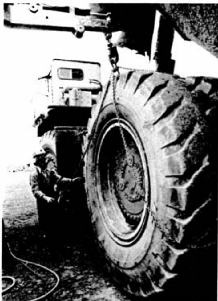
Changing a 42-ply tire on a 75-ton-capacity haulage truck requires special know-how. Here, United Tire's Tim Johnson rigs the tire with chains before lifting it with a mobile crane. Retreading will take place back at the shop.
