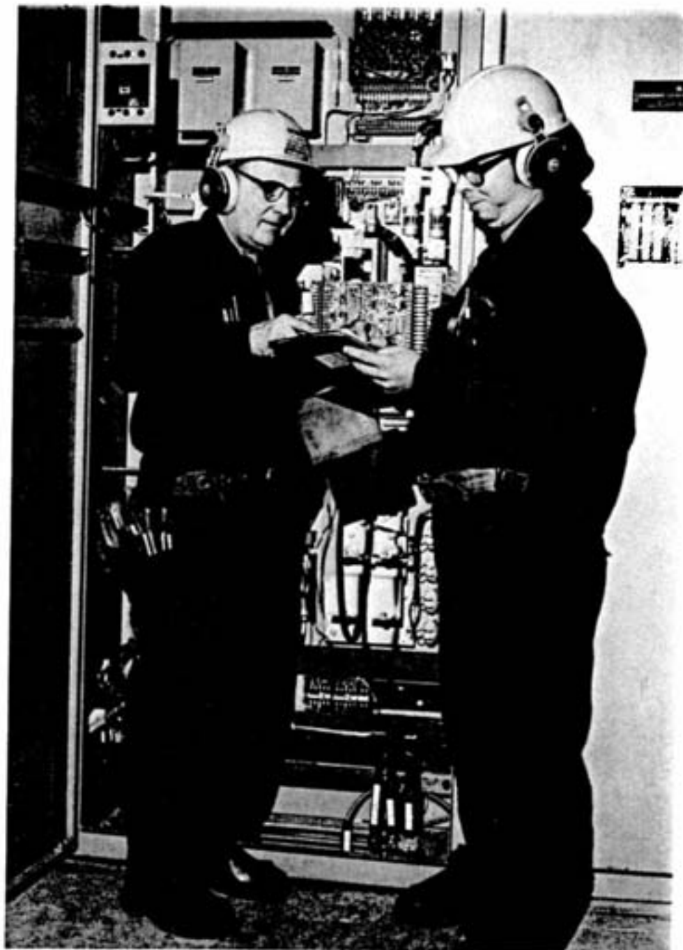
A solid state regulation and correction system for large synchronous motors was recently installed at the Levack mine No. 2 shaft skip hoist. Measuring the proper voltage on the system's power supply are electrician Al Cullis, left, and electrical foreman Tom Bayford. Incidentally, Al did much of the electrical work on the original hoist which was installed in 1954.
