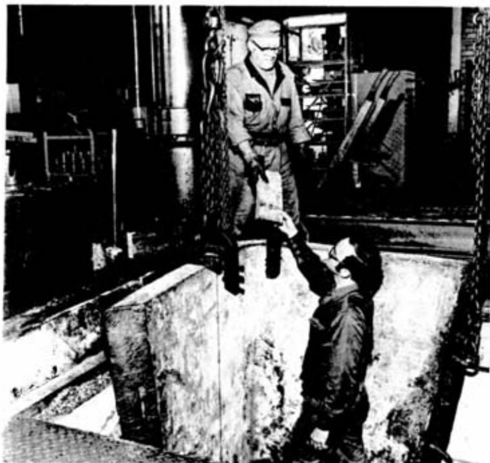
Gino Baldisera, top, and Michael Flood, both second-class maintenance mechanics, prepare to drill a water-cooled slag chute which is being repaired for the nickel reverberatory furnaces in Copper Cliff.
