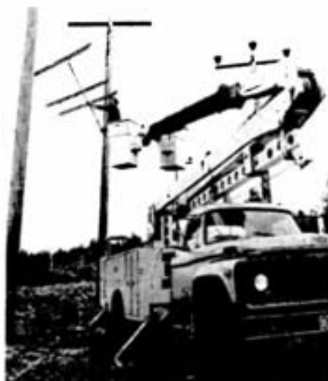
To ensure maximum safety, Delbert Merryiees, first-class lineman, installs insulating coverup on Ontario Hydro lines.
