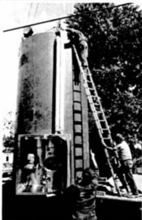
The Copper Cliff Dairy recently installed a new nickel stainless steel milk storage tank to further increase its milk storage facilities. The new tank holds 70,000 pounds of milk, roughly 7,000 gallons, and uses an ammonia cooling system to keep the milk at a constant 35°F. According to dairy manager Bill Johnson , the new tank doubles the storage capacity of the dairy. All milk processed at the dairy is obtained from local farmers.
