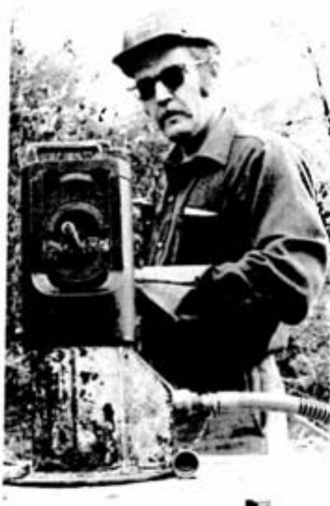
First-class lineman Lorne Kidd presses a sleeve on the 62-ton press, to connect the wires at the end of each reel to be strung.
