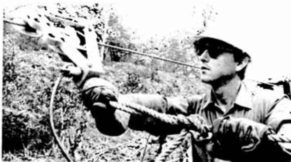
Glen Ganton, second-class lineman, installs a travelling ground on the wire that's being changed, to protect against possible contact with a live line. The job involved changing over 75,000 feet of wire.
