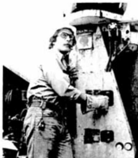
Gary Ackland, first-class lineman, controls the brake on the cable reel in order to maintain correct cable tension.
