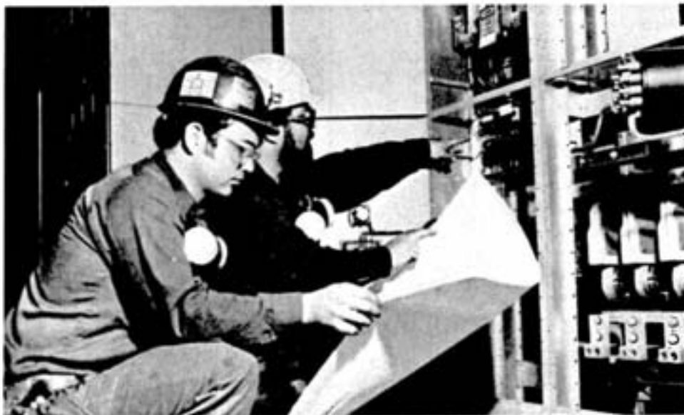
Water in the Orford Stack Cooling Tower is controlled from the Copper Cliff smelter's oxygen control room. Electrical gear located at the pump switch room provides operations staff with local pump controls and power. Apprentice electrician Kevin Robinson, foreground, listens closely as electrician Ray Newman explains the relay circuitry involved in the pump control system.
