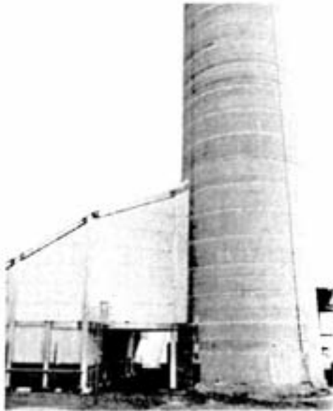
Located at the base of the 300-foot Orford stack, the cooling tower at left is the only one of its type in North America. Each of three cells is capable of cooling 6,000 gallons of water per minute from 160°F to 120°F.
