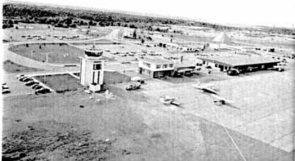
The Sudbury Airport complex, which includes control tower, administrative and weather offices, aeradio section and radio maintenance facilities, passenger and cargo-handling facilities, and maintenance buildings.
