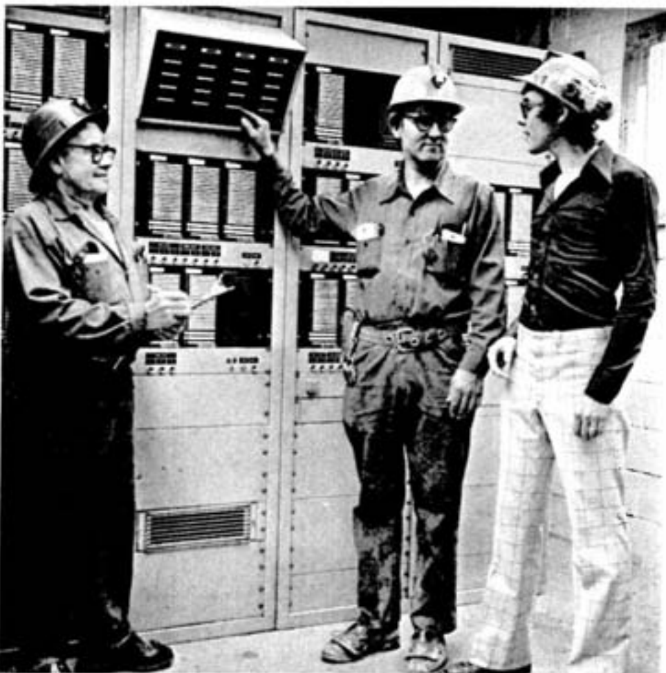
The Modudata system at Creighton mine automatically indicates which pieces of stationary underground equipment are running and at what capacity. Operating shaft boss Rolly Richards, left, listens in as electrician Leo Laakso reads a pump current readout to Everett Henderson, right, electrical technologist.
