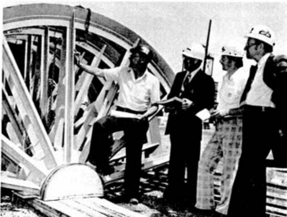
Recently arrived from England, these sheave wheels are scheduled for installation in the Garson mine headframe this summer. Prior to their installation, the wheels receive a thorough inspection by, from left, Fern Dionne, Garson mine zone planner; Largo Albert, hoisting specialist; Dick McIvor, design engineer, and Ted Tuori, Garson area maintenance superintendent.
