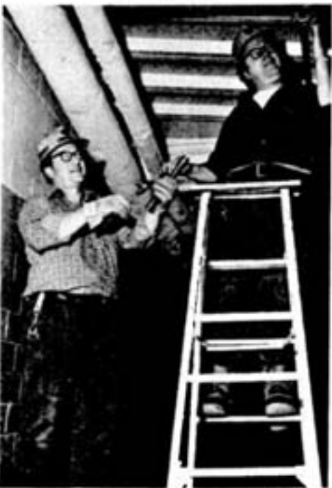
Renovations at Creighton mine's No. 3 shaft included the construction of a new training centre on surface. The training centre will provide personnel with a central location to study maintenance techniques. Here, maintenance mechanics Yogi Bjerknes , left, and Jim Stefanko install the centre's air line, designed to supply compressed air for hand-operated tools used in the training program.
