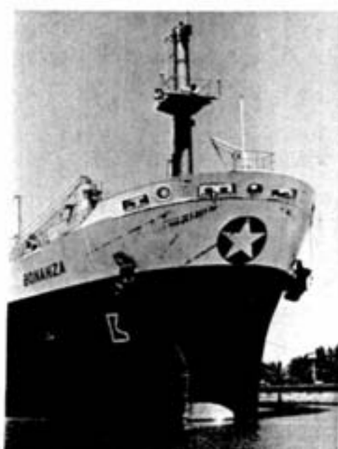
It takes only eight to ten minutes to fill a lock with about 25 million gallons of water, raising a ship 46½ feet. Depending on the number of other ships encountered, it takes eight to ten hours for a ship to pass through the 26.7-mile-long Welland Canal.
