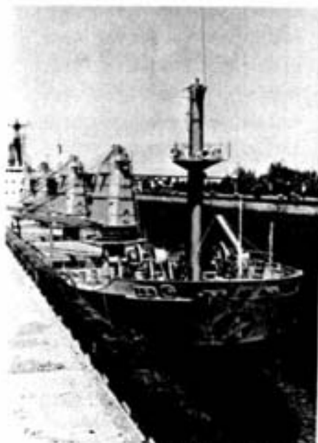
It takes only eight to ten minutes to fill a lock with about 25 million gallons of water, raising a ship 46½ feet. Depending on the number of other ships encountered, it takes eight to ten hours for a ship to pass through the 26.7-mile-long Welland Canal.
