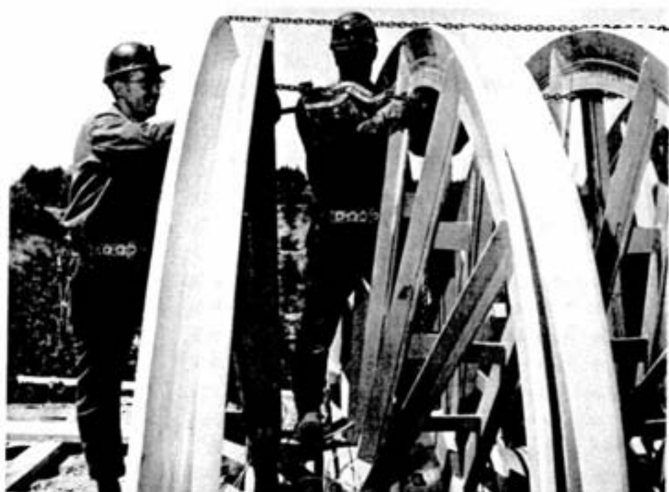
Bisected for easier transportation, the sheave wheels will be bolted together at the rims, and a heated shrink ring will lock the sections together prior to installation. Before these procedures can take place, riggers Leo Deguire, left, and Lloyd Cowper "beartrap" the sections to prevent them from falling over. Each of the sections weighs 4,171 pounds.
