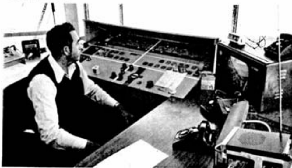
From a single control tower, all facilities in the vicinity of Lock No. 8 can be operated and watched. Two closed-circuit television monitors help determine when ships are clear of lock gates and bridges, which helps speed the ships through the lock.
