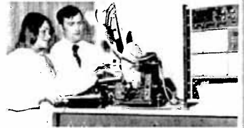
Inco's process technology laboratory in Copper Cliff is extensively involved in an occupational monitoring program involving analysis of air samples from area mines and surface plants. Free silica in airborne dust is collected with a personal monitor filter which is analyzed using the X-ray diffraction spectrometer, shown above, which gives a numerical printout of the X-ray intensities. Shirley Lowe , summer student, and section leader Stan Maggs insert one of the filters into the machine which is proving highly beneficial.
