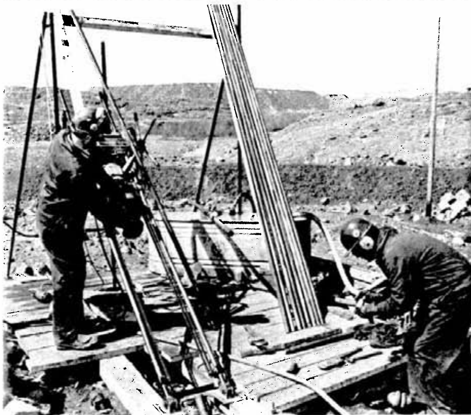
Inco's field exploration department in Copper Cliff recently tested their newly modified "Super Winkie" diamond drill on site at the Clarabelle open pit. After successfully completing a 200-foot hole, drilled at a 45° angle, it was found that modifications had doubled the original capacity of the drill. Here Keith Allen , left, drill supervisor, and Lawrence Kearney , drill runner, are getting ready to pull another "A" steel rod from the hole.
