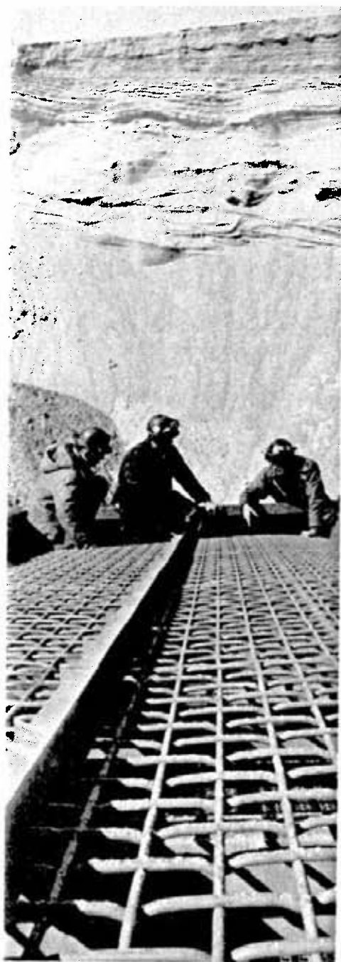
A bird's-eye view of the new mobile screening facility at the Garson sand pit. Adjusting the unit are maintenance foreman Gerald Hinds, left, and maintenance mechanics Don Morin and Don Milbury.
