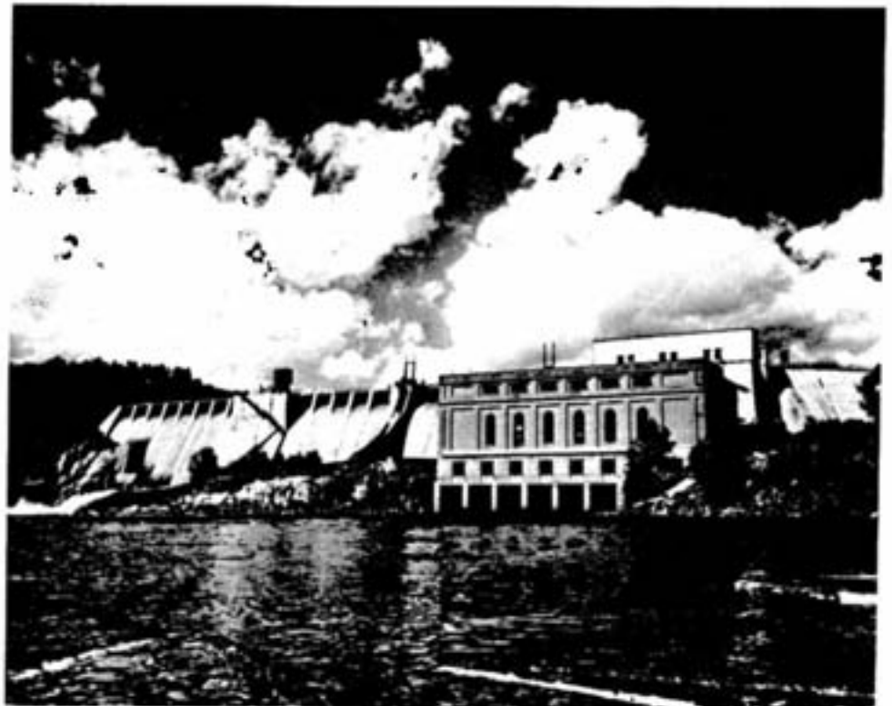
This is the Big Eddy Power Plant, one of four on the Spanish River. Built in 1928, it is the largest, with a generating capacity of 24,500 kilowatts.
