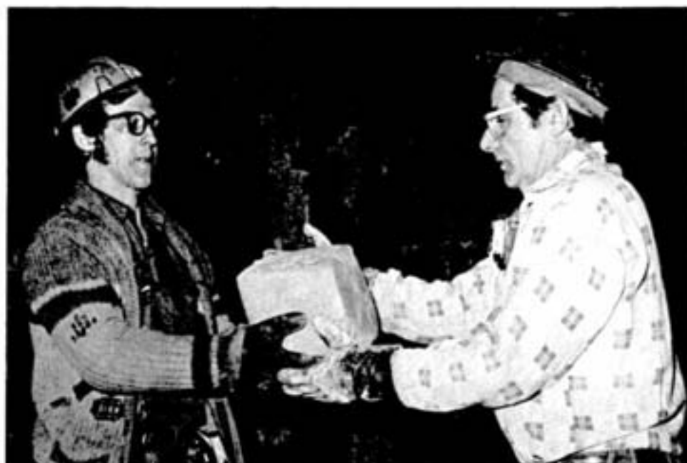
Shaping fire clay for use in budding up matte tap holes are clayman helper, Gerry Larade, left, and clayman Gerry Niehoff. The fire clay, which will be distributed to the tappers, can easily handle the 2,200°F. temperatures of matte from the reverberatory furnaces.
