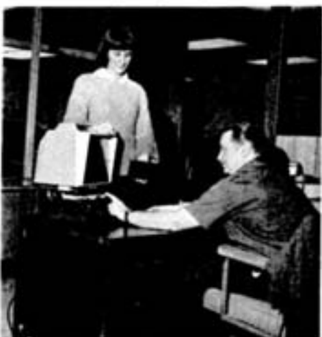
This is a microfiche viewer which provides an accurate and compact method of reviewing inventory. Used as a replacement for the bulky master catalogue, a computer printout, the viewer can project the enlarged image of microfilm slides onto a viewing screen. Three of the old books can be condensed onto 23 microfilm slides. Vic Lumbis , a materials controller with inventory control, scans the slides, one of which is held by Frood-Stobie maintenance clerk-stenographer, Shirley Sasseville .
