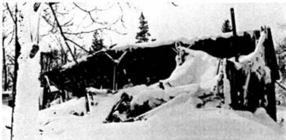
This barn in the township of Wainfleet just couldn't take the weight of snow and collapsed.
