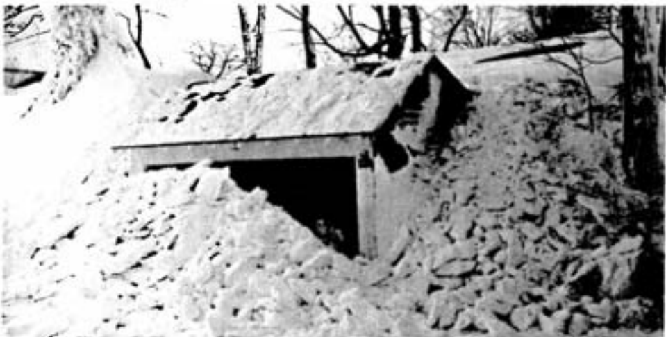
This garage was almost totally buried in snow and probably would have collapsed if the owner hadn't removed the snow from the roof.
