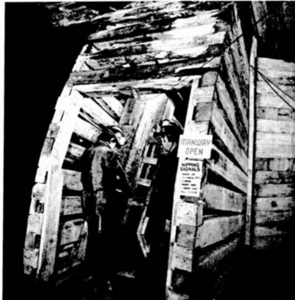
One of Copper Cliff South mine's unique features is this cribbed raise used strictly by the school stope where novice miners are familiarized with nipping procedures. Here, Royce Blackwood, training supervisor, checks the nipping procedure of shoveller Ray Stephenson. Nipping involves the proper method of moving material from one underground level to another.
