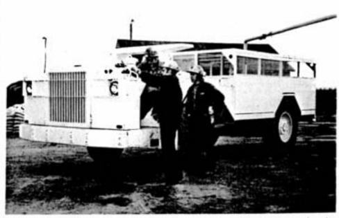
Equipped with a 180 horsepower Caterpillar V-8 engine, this new 24-man personnel carrier will be moving miners between surface and the 1725-foot level of Creighton mine's 3 shaft ramp. Below, training supervisor **Wilf Little**, right, instructs boom-truck operators **Augusto Ferri**, left, and **Lawrence Martin** on the operation of the vehicle.
