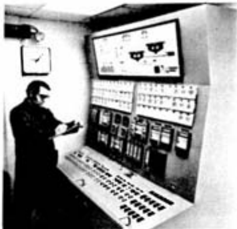
The control console at the new water treatment plant, which also monitors operations at the Nolin Creek plant in Sudbury.
