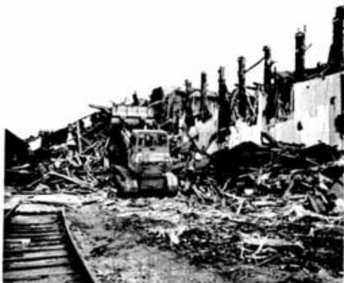
The wrecking contractor's bulldozer clears rubble from the ore bins. These wooden structures are hundreds of feet long and were used for bulk ore storage.
