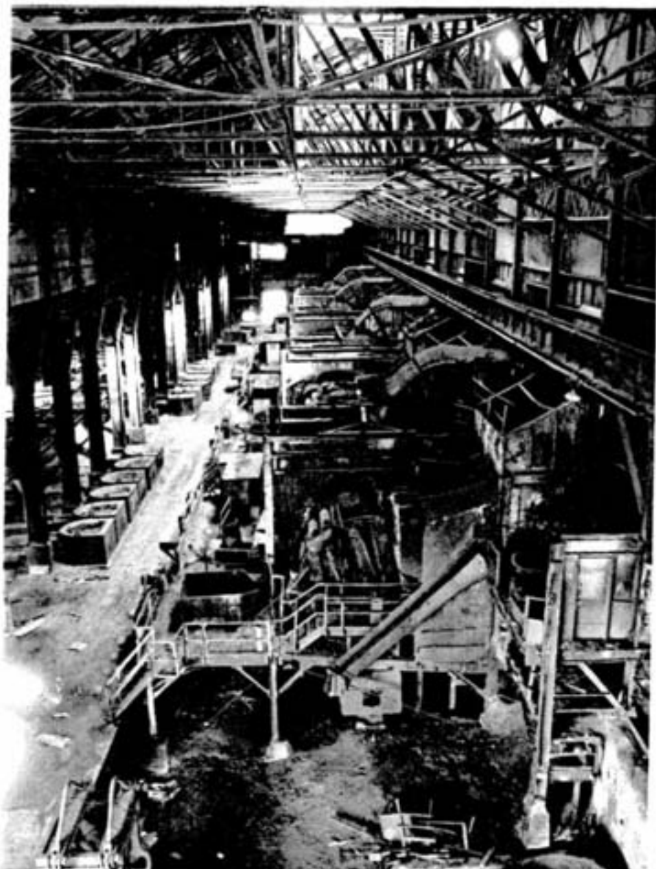
The main converter aisle in the Coniston smelter sits idle, awaiting the wrecking crews. The four converters poured out their product around the clock until 1970, when the smelter was closed. Rails along both sides of the structure supported the overhead crane, which ran the full length of the building.
