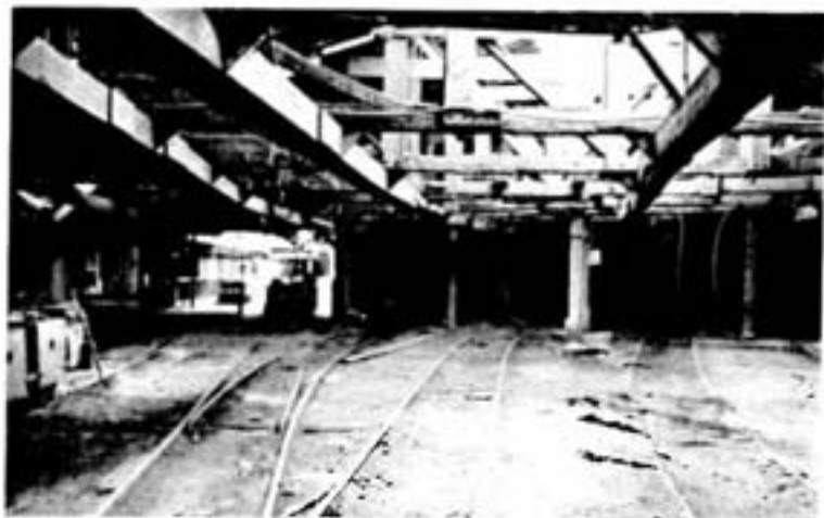
This is a view of the charge trestle from the inside, showing part of the locomotive repair area. The major portion of the structure was composed of huge timbers.
