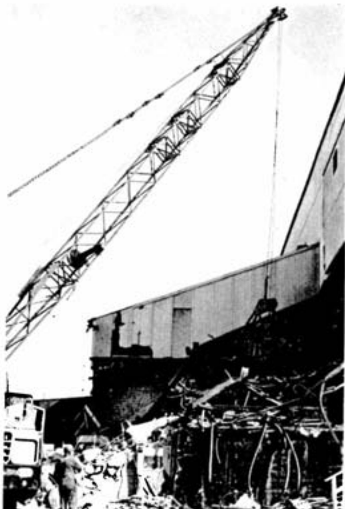
With the big crane in action, it doesn't take long to rip apart steel siding from the converter building. The structure, built in 1912, was originally owned by the Mond Nickel Company.
