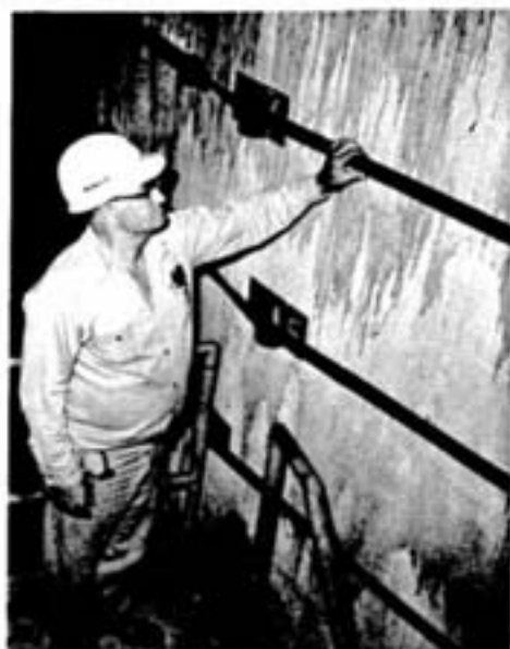
Extensive repairs were recently completed on the main ore silo at Creighton mine. The silo, which handles all ore from Creighton number nine shaft, was relined with rails along its inner walls. Also, the outside was banded with 3/4-inch diameter steel bands, tensioned to 48,000 lbs. each. Here Creighton mine services foreman Andy Ostashek examines the outer banding of the silo which has a holding capacity in excess of 3,000 tons.
