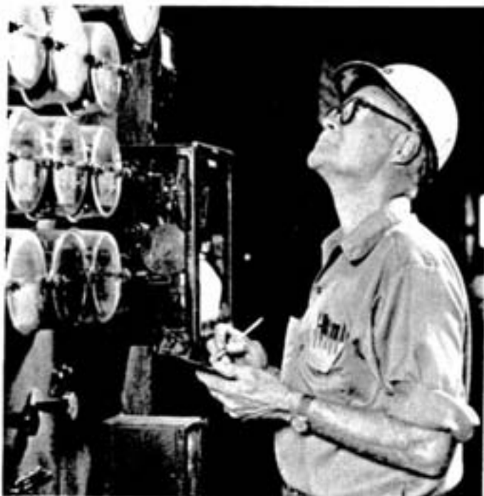
Substation boss, Gus Carthew, takes a reading of the load and incoming voltage at the new south substation. The electrical power is recorded on the meters before it enters the power converters.
