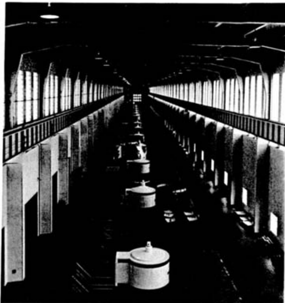
A view of the 16 turbines at the Sir Adam Beck generating station number two. This station produces 1,400,000 kilowatts, more than half of the energy produced by Ontario Hydro at Niagara.
