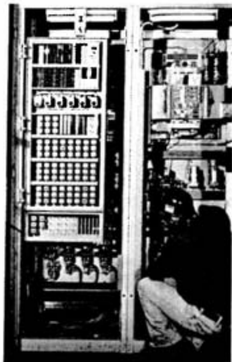
Gerry Stokes, first class electrician, inspects solid state control cubicle.
