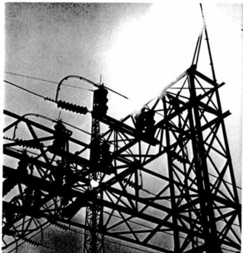
The Davis Street transformer station. A voltage of 115,000 volts is carried by high-tension wire to the station from Niagara Falls. It leaves the station at 27,600 volts before entering the converters.
