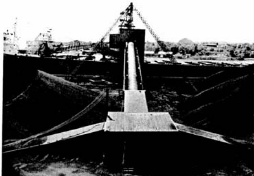
Iron ore pellets at the Little Current dock are transported by conveyor system, left and right, to the main conveyor in centre. This in turn carries them into the ship's hold.
