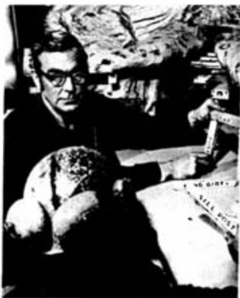
Through the use of blocks, instructor John Chivers explains the drift timbering techniques used in modern mines. According to John, the use of these blocks has done much to simplify instructions.
