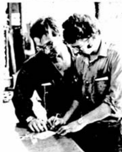
Keeping safety in mind, garage mechanics Richard Maskevich , left, and Jim Russell sign a personal protection tag. The mechanics, who work at the Levack West mine, sign the tags and hang them on the starter controls of machinery they are working on to show others that the equipment is still under repair. The personal protection tag is a common sight at all Inco operations.
