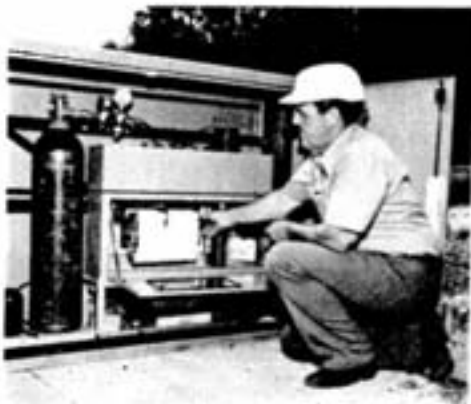
Shebandowan mine engineer Bill Allard checks a flow meter located on the Matawin River, twelve miles downstream from the Shebandowan mining complex. The flow meter is designed to indicate the amount of water that flows over the tailings dam and into the natural watershed. Information obtained from the unit allows for control of water flowing from the pond.
