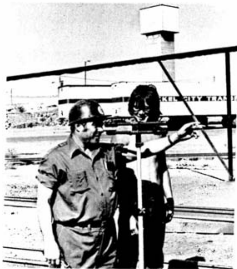
Learning from a real pro, summer student Dave Rochon listens while track foreman Joe Longhi describes a section of track that needs to be repaired. Joe is lining the track with a scope which indicates warps that can be corrected with the help of the track liner.
