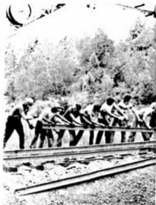
Teamwork is essential in laying rail, and Inco's extra gang down a few more yards of track while track boss Fra seated correctly.
