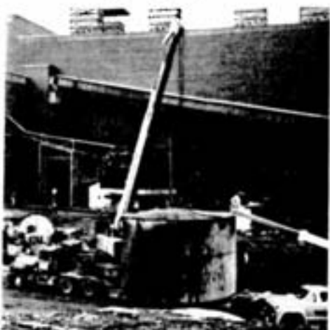
Moving an oil storage tank 14 feet high and weighing some 15 tons is no easy undertaking, even for Inco's transportation department. The tank was recently moved from the smelter complex to the iron ore recovery plant storage area. A 25-ton float and a 55-ton crane were required for the move, and a line truck was called in to raise wires along the route. Welders were required to remove gateposts at one of the plant entrances to allow passage of the 20-foot-wide tank. The move was supervised by Bob Burke of the Copper Cliff transportation department. Vic Henderson and Les Cresswell assisted in the move, along with an escort by the Sudbury Regional Police and a CPR flagman stationed at level crossings.
