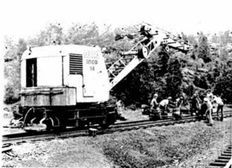
Giving the extra gang a boost, a crane is used to mount a rail cutter on the track. The rail cutter is used to take out worn sections of track which will be replaced with new steel to ensure a safe foundation for passing trains.
