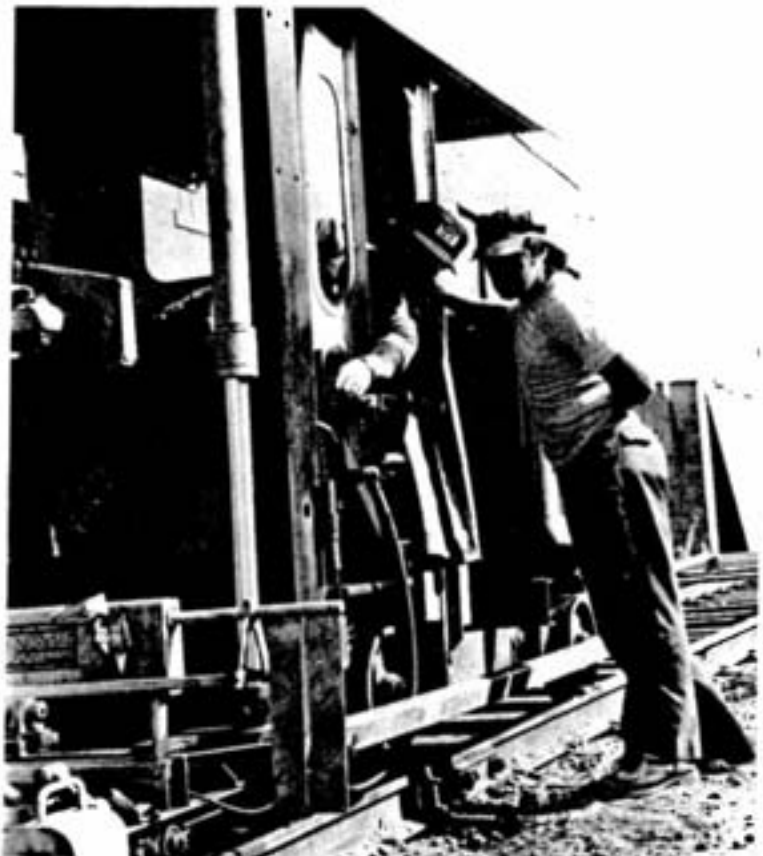
Track liner operator Danny Brazeau explains to trackman Don Alexander how the machine registers a warped rail. A beam of light is passed from the front of the track liner and is picked up by an infrared receptacle at the rear. If the beam is uninterrupted, the track is straight.
