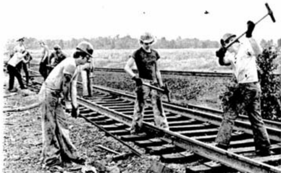
Using muscle power to get the job done, extra gang workers Dan Imbeau, Ken Graham and Ido Vettoretti pound spikes along Inco's 100 miles of track. During the summer, eight crews take a section of up to 12 miles for necessary repairs and renovations.
