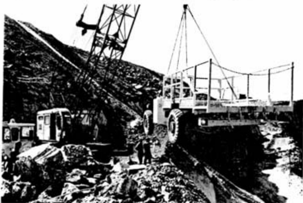
This scissor lift truck was recently lowered over the wall of the Froid Open Pit to a portal in the pit wall and driven down an internal ramp to 800 level. According to maintenance general foreman Bob Conlon , a crew of six riggers performed the job in only four hours! Scissor lift trucks are utilized underground in numerous operations, such as roof bolting, screening, pipe hanging, scaling, explosives loading and carrying supplies. It can also double as a personnel carrier when fitted with optional fold-up seats to carry 14 men.
