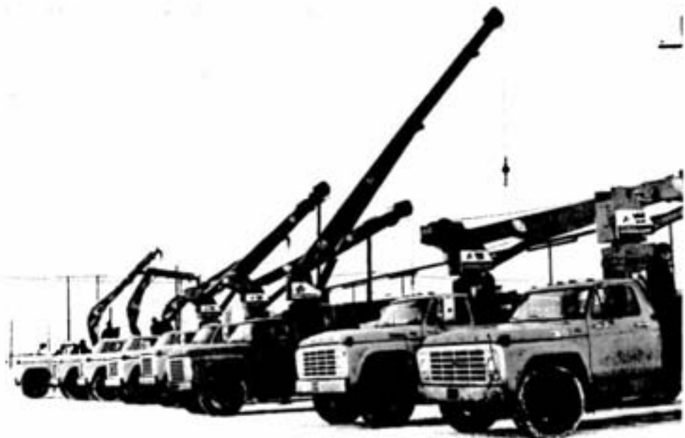
That's Inco's fleet of lift trucks, operated by the transportation department in Copper Cliff. Boasting an average lifting capacity of 6 to 7 tons, the trucks are sent to different plants and mine sites from the dispatcher's office. For a more efficient operation, a number of the units have been equipped with two-way radios. The skilled operators are, from left, Roger Spencer, Pete Parisotto, John Turner, Walter Precholko, Walter Pihursky, John Berube, Felix Lalonde and Reg Lamirande .
