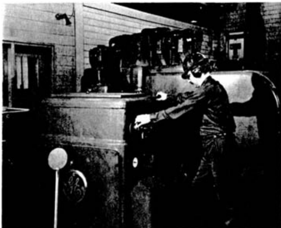
Second class stationary engineer Ben Munch makes final adjustments to the speed control of the steam turbine generator at the Iron Ore Recovery Plant.
