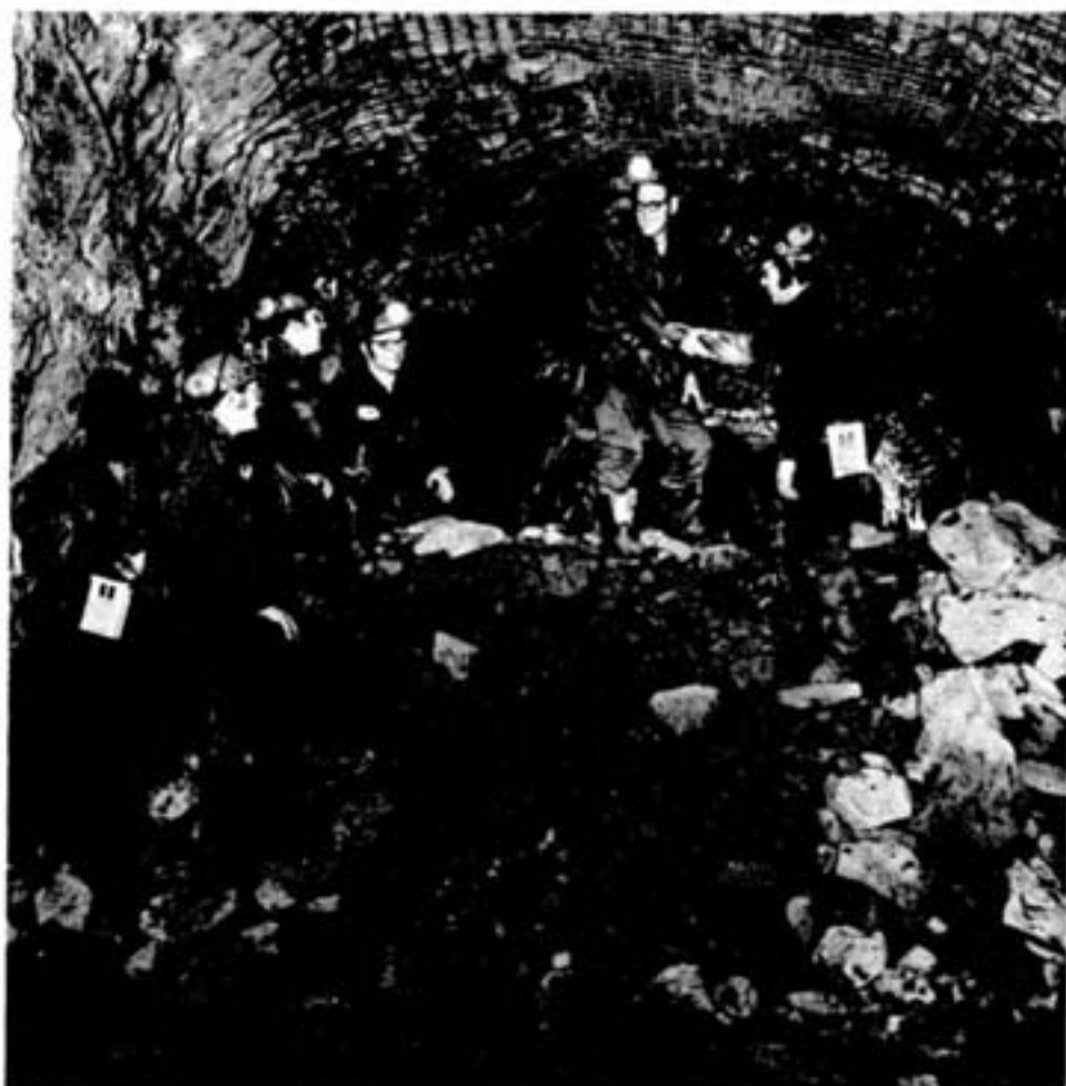
Development crews recently blasted the final round of the Little Stobie to Stobie mine sandfill drift, some 3917 feet in length. Driven from both Little Stobie and Stobie mine on the 600-foot horizon, the drift measures 11'6" x 12' in diameter and will provide sandfill for Little Stobie mine. Congratulating each other after the final successful blast are, from left, Raymond Laurin , diesel loaderman, Little Stobie; Wayne Casy , jumbo driller, Little Stobie; Gerry Brouillette , driller, Stobie; Gaston Beaulieu , jumbo driller, Stobie; and Tom Lacroix , driller, Little Stobie.
