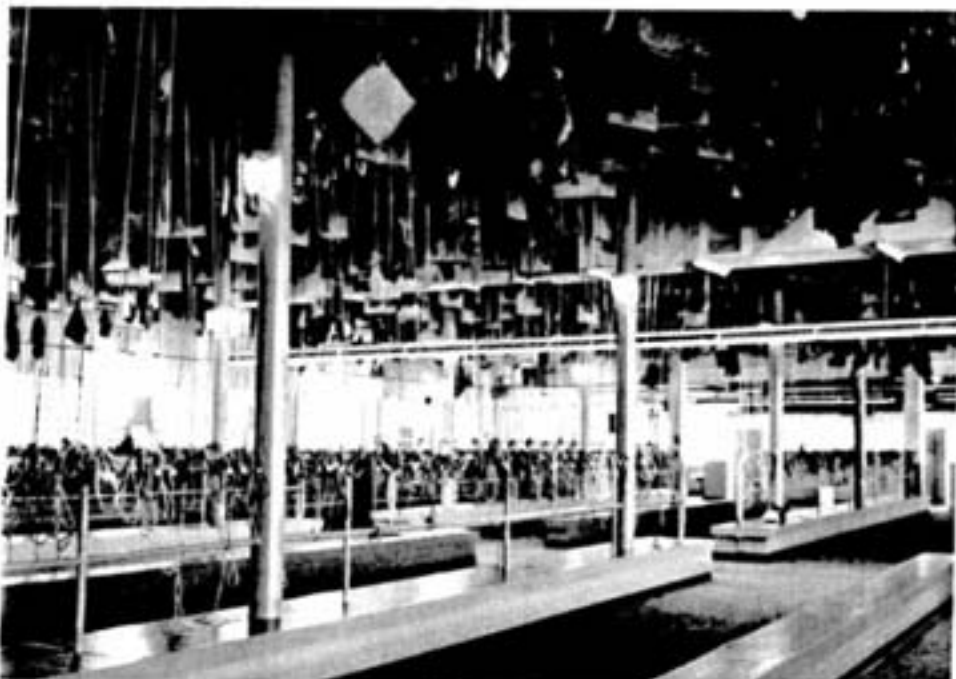
Number three changehouse with its lofty ceiling and rope lockers. One of the important features is that the clothes are well ventilated.
