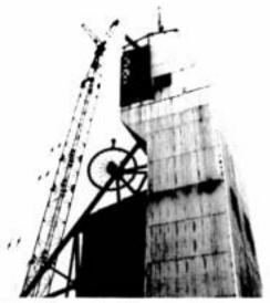
One of the new head sheaves, weighing 8 tons, is being hoisted to the top of the 163-foot headframe, using a 60-ton crane.
