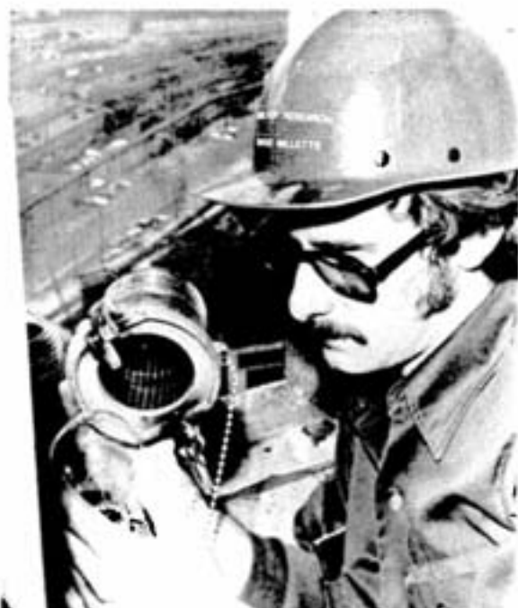
336 feet above ground level, at the stack's second service platform, Dave Mallette, project assistant, smelter process technology, swings in a pair of aircraft warning lights for a closer look. There are 48 such pairs, strategically located up, down, and around the stack.
