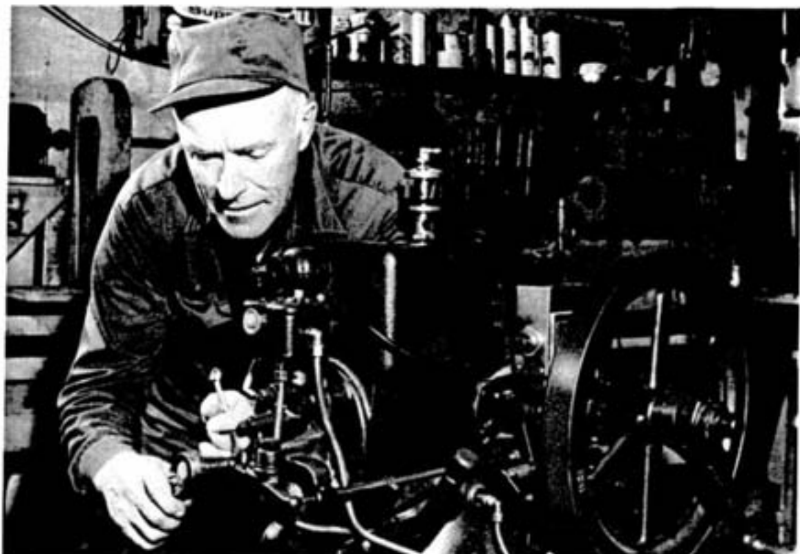
In his basement workshop, antique engine restorer and Inco pensioner, Ken Weaver, makes final adjustments to a rebuilt International Harvester one-and-a-half-horsepower gas engine that was built in 1919 and now looks like new
