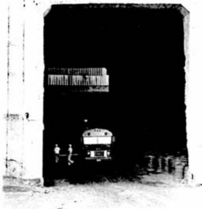
Travelling the road that passes through the base of the superstack, an Inco tour bus pauses to unload passengers for a look inside the huge "cavity" — there's enough room inside to park over 250 cars! The photoelectric cell to the left of the entrance automatically activates the stack's lights from dusk to dawn.
