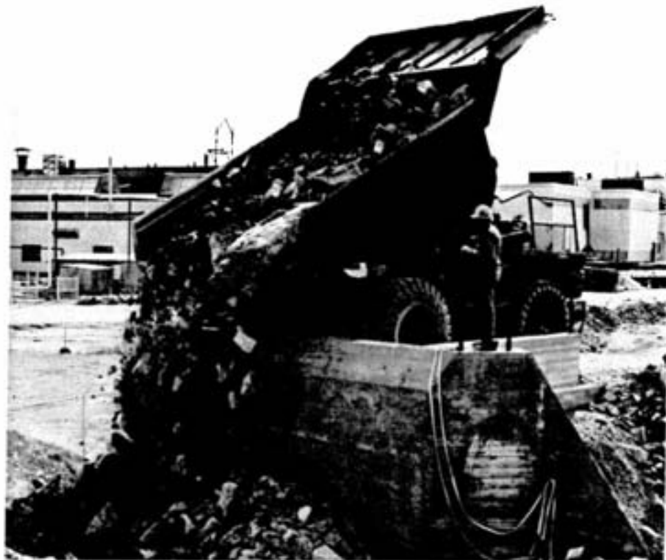
Another load of rock, 35 tons' worth, is dumped down a raise bore hole at Copper Cliff South mine. The rock free-falls directly to the 500 level where it is used for fill in underground mining operations. This method of delivering rock from surface is very efficient, and is one way that Inco can make use of waste. Observer is foreman Herman Woltman.
