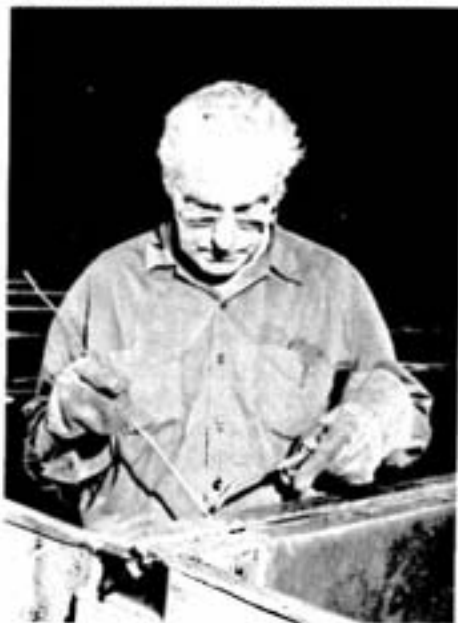
Lead welder, Jim Smith, at the Copper Cliff copper refinery, puts the finishing touches on one of the newly installed lead linings.
