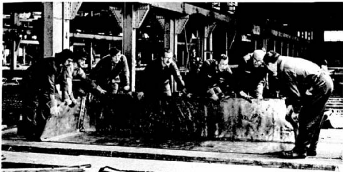
After forming the lead sheet on the dressing platform, this crew attempts to position it for removal by the overhead crane. Men are, from left, Pat Hudson, George May, Mirko Dobrich, Marcel Labelle, Joe Burns, Charlie Martinu and Sam Budzak.
