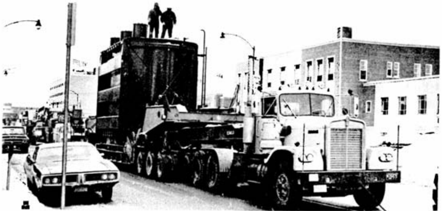
The 150,000-kilowatt transformer en route to the number four sub-station at Copper Cliff. The 112-ton load was moved nine miles at a maximum speed of four miles an hour. The float was 108 feet long, and the loaded transformer towered 20 feet above road level.
