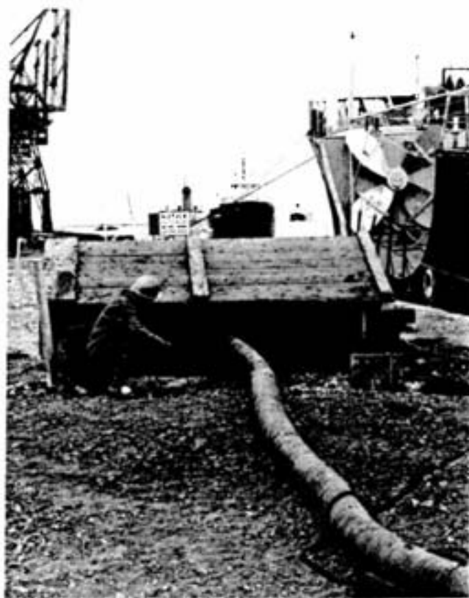
A very thick oil, bunker "C" is heated on-board to about 125°F. At that temperature it flows freely and can be handled by on-shore pumps.
