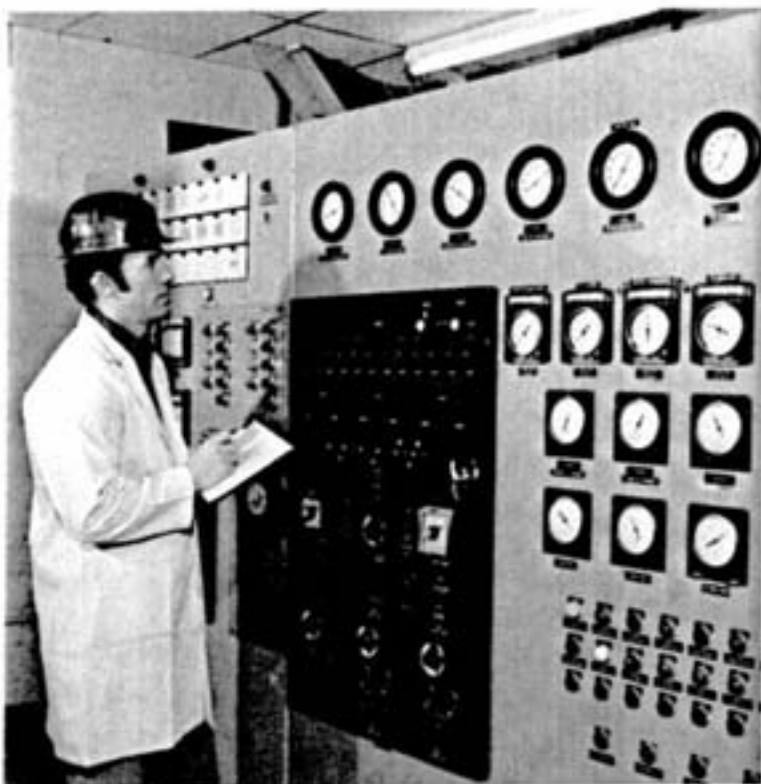
Gary Bradley, Inco oxygen plant operator, monitors flow of krypton from main control panel at oxygen plant. All phases of Inco's oxygen plant can be controlled from this area.
