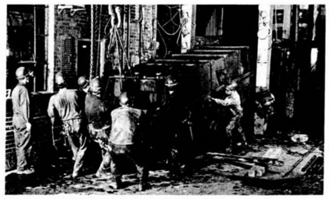
Under the direction of maintenance foreman Ed Luoma (left) riggers remove one of the mine's two existing bottom-dump skips. The skip weighs 10 tons, with a capacity of 247 cubic feet.
