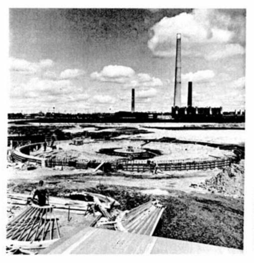
The purpose of the Copper Cliff creek plant, which is being built in the best possible location to catch the waste from the smelter, is two-fold; to clarify the waters of the creek and the waste from the smelter and, at the same time, to reclaim any of the concentrates which may be flowing in the creek.
