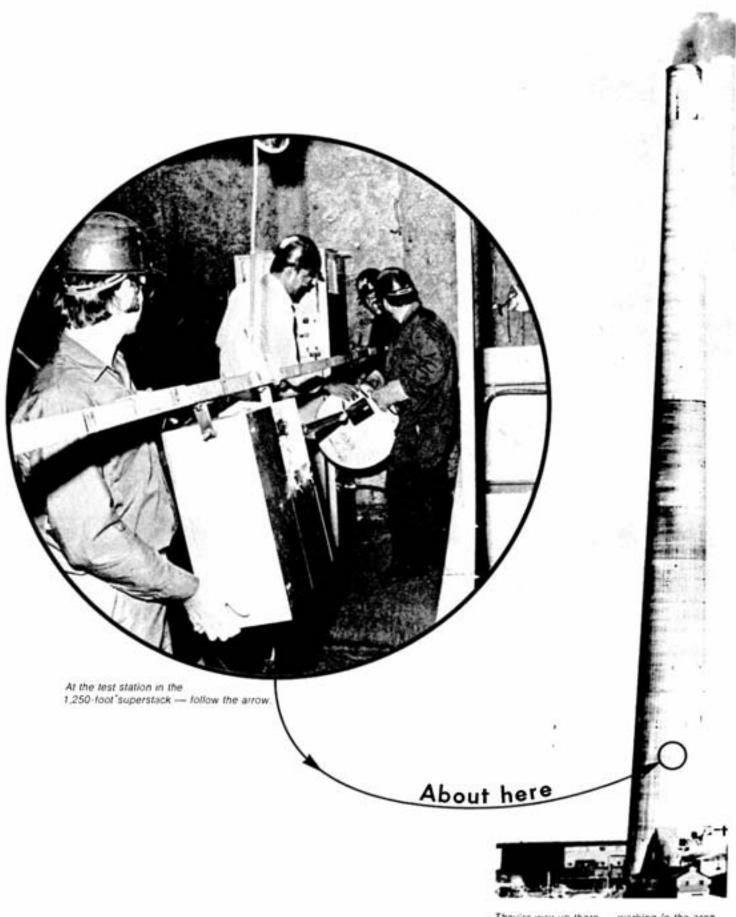
They're way up there — working in the area between the concrete stack and its steel liner.
