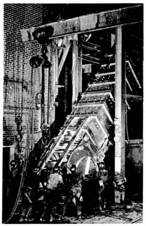
Tipping the scale at nearly six and a half tons, a glearning new roller gate type skip is eased gently into the shaft. It has a capacity of 290 cubic leet.
