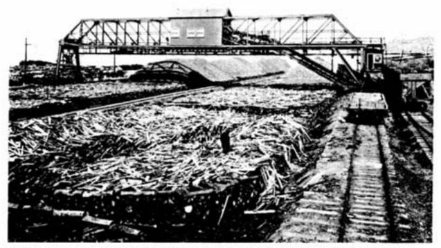
Individual roast beds were 100 feet long by 60 feet wide. With a clear span of 170 feet, the travelling green ore unloading bridge serviced the mile and a quarter long roast yard. On the average, a bed burned for seven to eight months.
