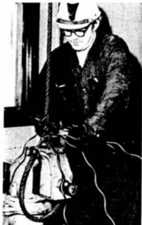
Rigger Don Spurr splices a 3/4-inch cable sling with a 36-inch eye. To a rigger, wire slings for lifting are as important as a lariat to a cowboy.
