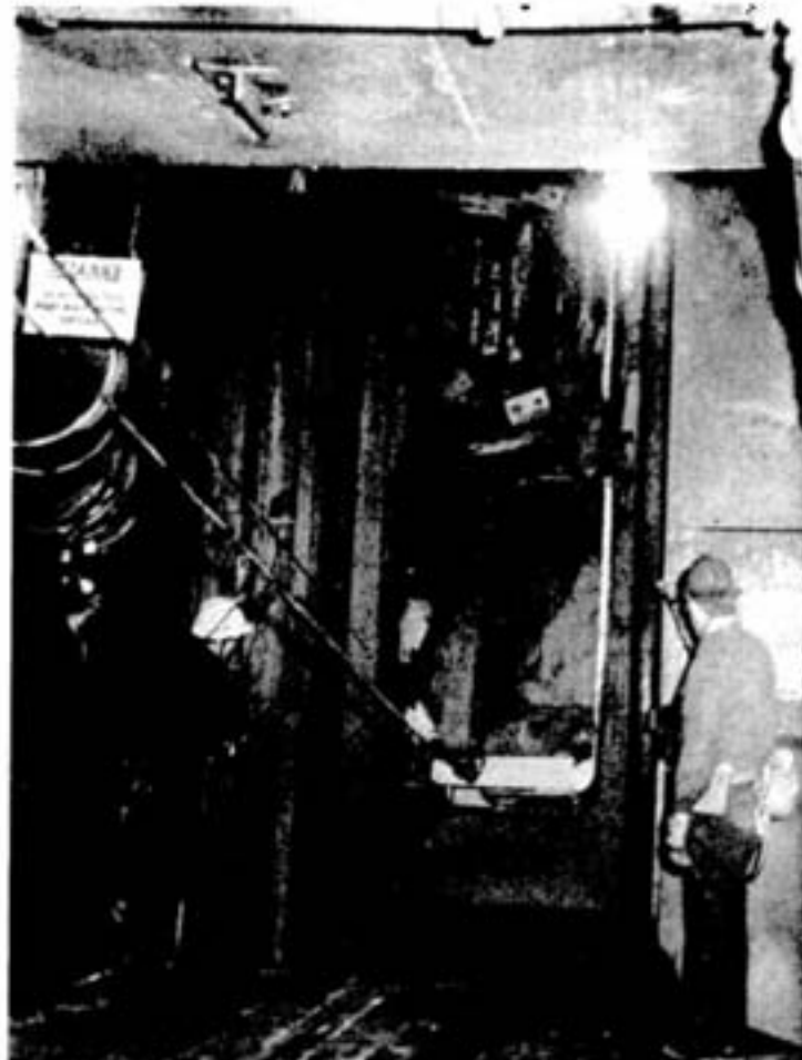
On 6600 level, Bill Blackwell handles the hoist signals as the machine is slowly lowered and drawn out onto the station deck by a tugger hoist. Note the more confined work area. The other riggers are John Melanson and Gordie Golden.
