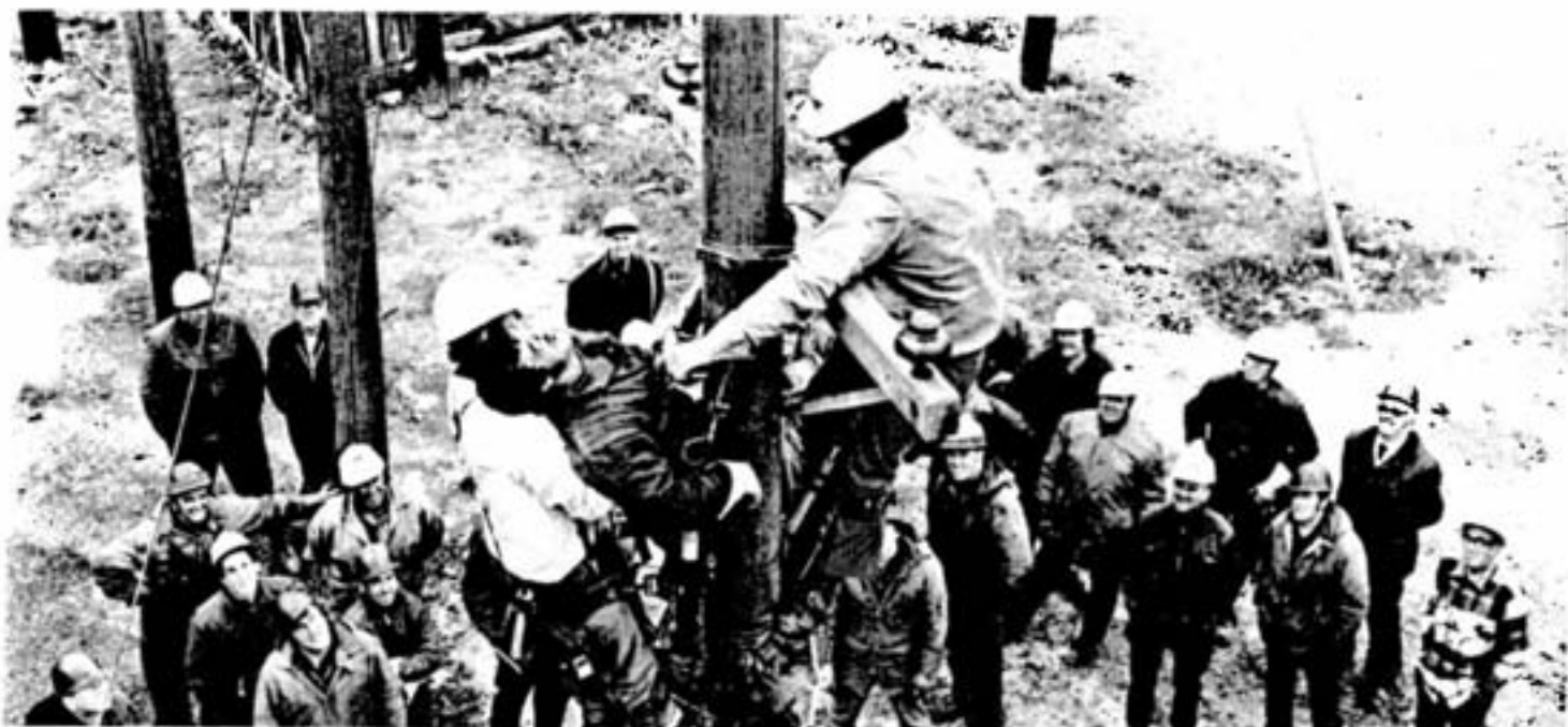
The demonstration "victim", Reg Campbell, hangs limply from his pole belt while Cy Gravelle places himself in position to apply a form of artificial respiration. Inspector Tallon prepares the rescue rope to lower the "victim" to the ground. Inco line and telephone crews watch intently.
