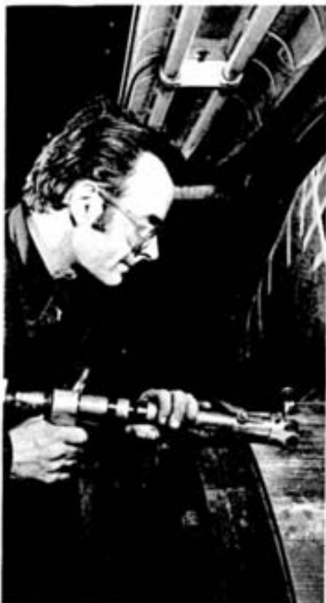
Mica, the insulation between the commutator's 1,340 individual copper conductors, was trimmed down by "Pinky" Pilkington.
