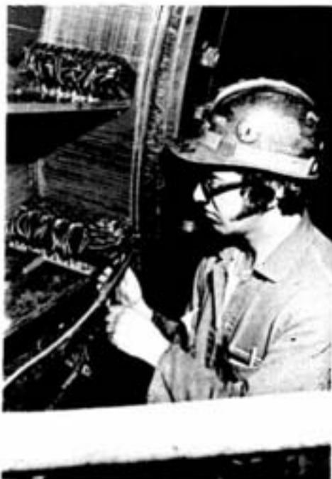
One of the final steps of the job, the re-installed brush rigging was adjusted by maintenance electrician Dan Gagne.
