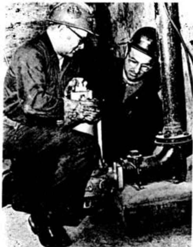
A 14-foot deep wet well includes two pumps, here installed by Bernie Forestell (left), and Frank Sottile, that lift influent to the clarifier.
