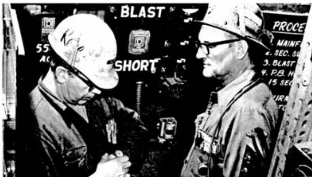
With blast zero-hour just seconds away, area electrical foreman Rene Plouffe counts-down for mine foreman Eric Ashick who triggered the blast. Using mains voltage, the switch activated a circuit breaker and 14 loco batteries on the 600 level which provided the 600-volt DC firing jolt.
