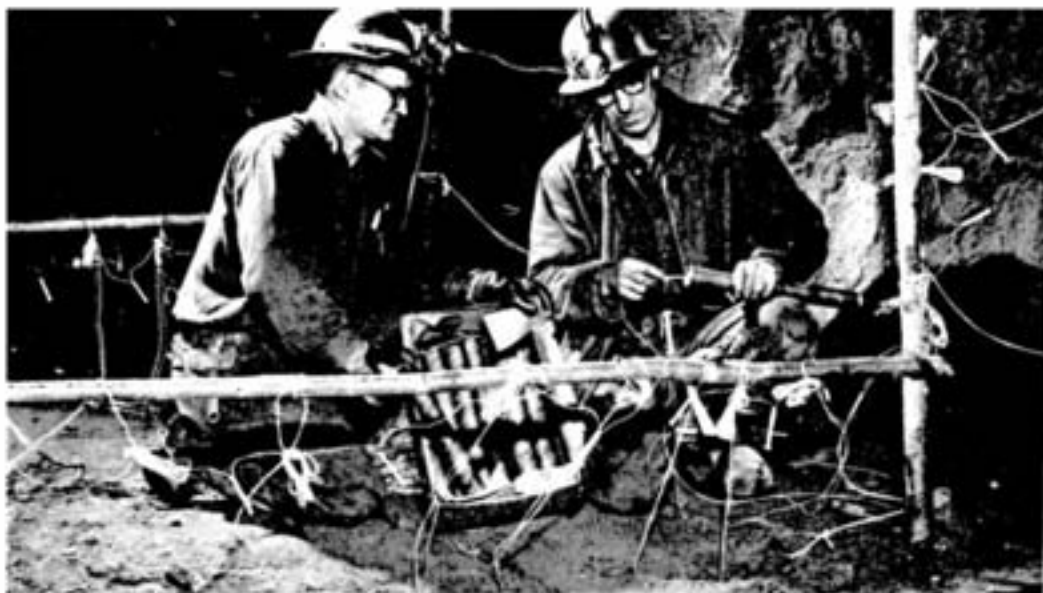
At the south end of the 120 orebody and on the 400 level, construction leader Don Cucksey (left) and blasthole drill boss Fred Monette re-prime a drill hole in the main north drift. Except in wet and lost holes, stick powder was used.
