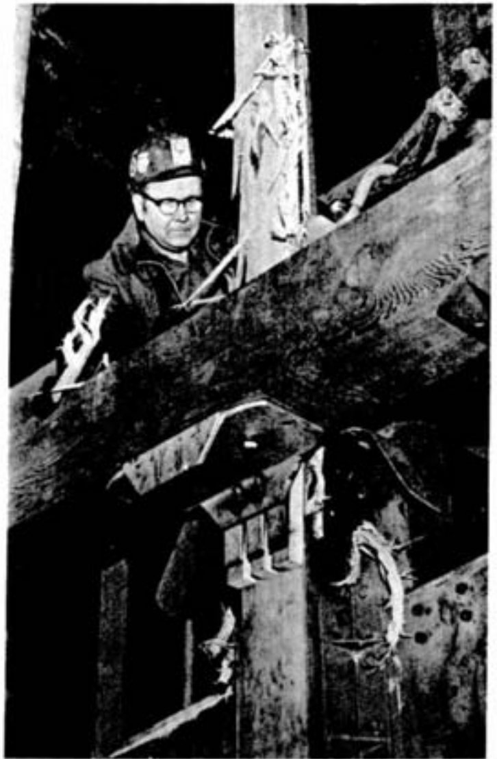
This is what happens when the dogs are released. Maintenance foreman Floyd Kennedy examines one of the four pairs on each cage. Note how deeply they bit into the guide. In this test the cage stopped in 4.85 feet.
