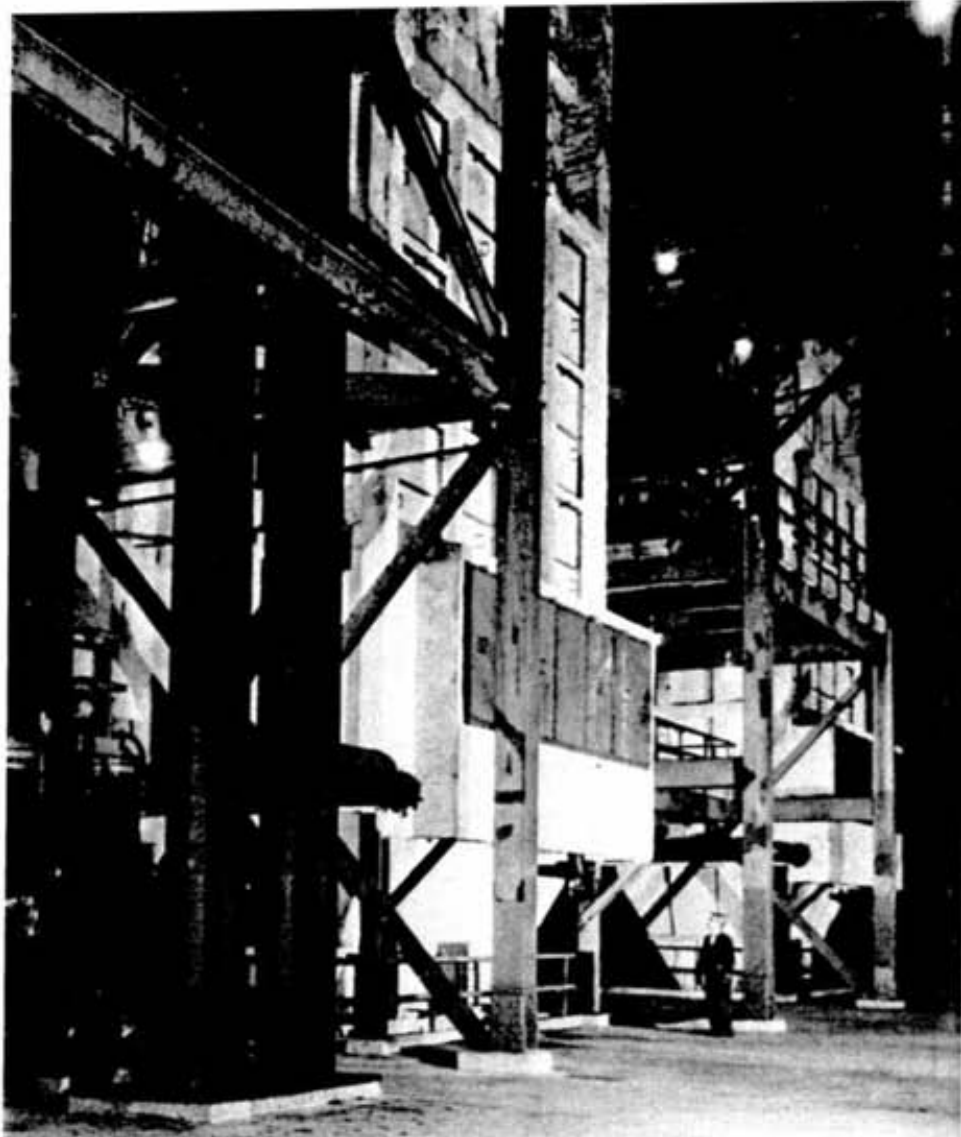
Six waste-heat boilers at the iron ore recovery plant develop steam, using heat from the fluid bed roasters, for plant heating and electricity — enough to power a city having a population of 20,000.
